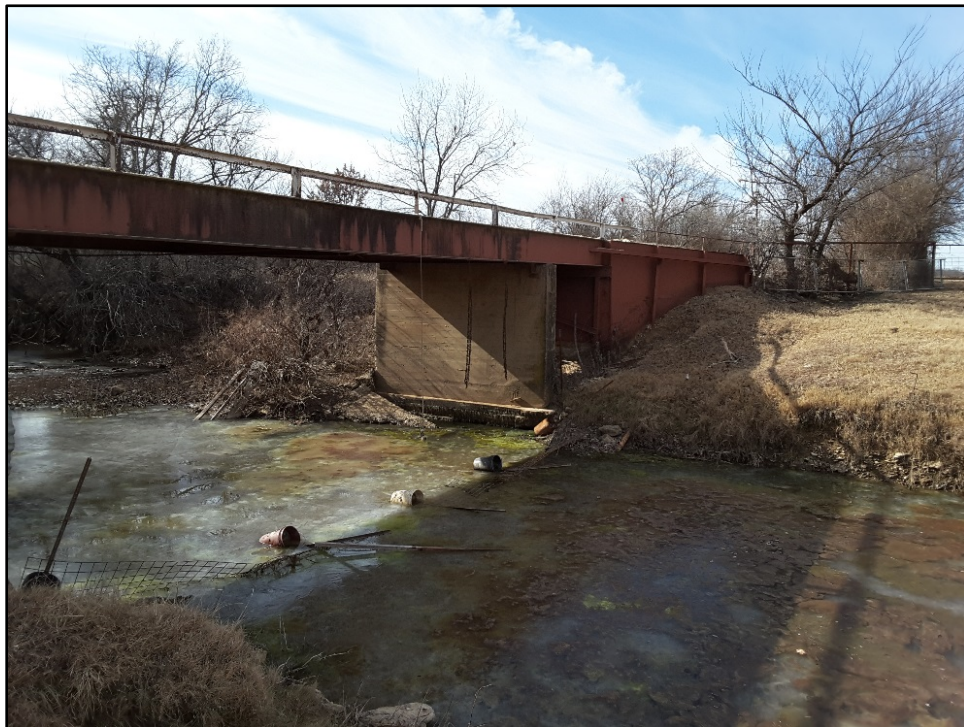
Figure 7. Temporary easement on northern side of APE.
