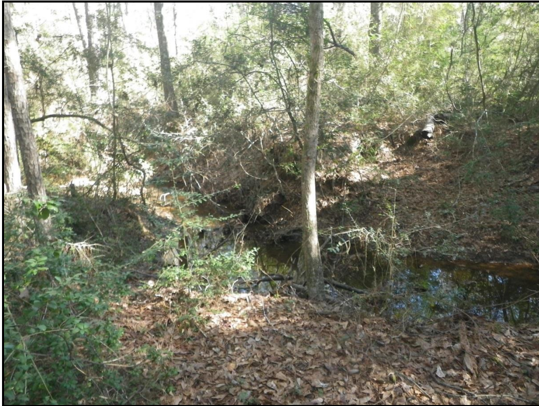
Figure 7. General photo of the northern detention basin area, including an intermittent creek, facing west.
