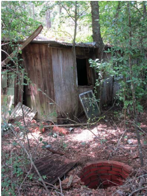
Water well on northeast corner of the building
