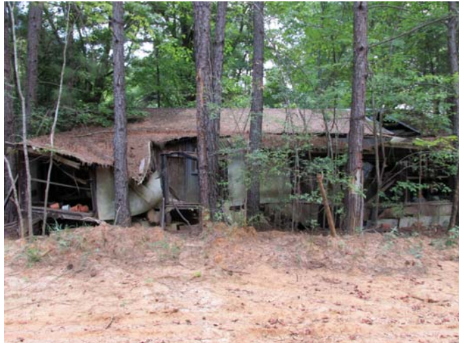
South elevation of building (looking north)
