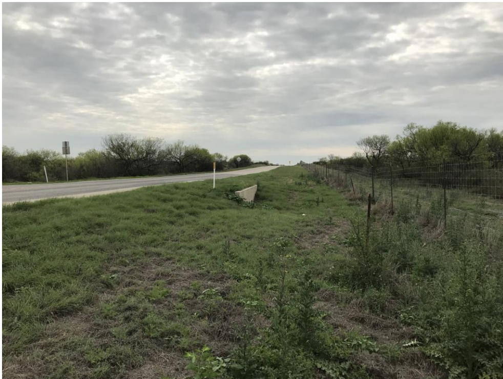
Typical FM 186 culvert replacement ROW in central portion of APE.
