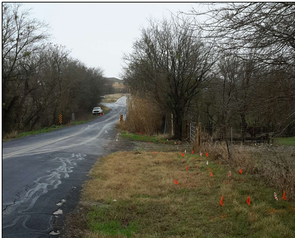
Figure 3. Narrow ROW showing marked utilities on both sides of roadway, facing south.
