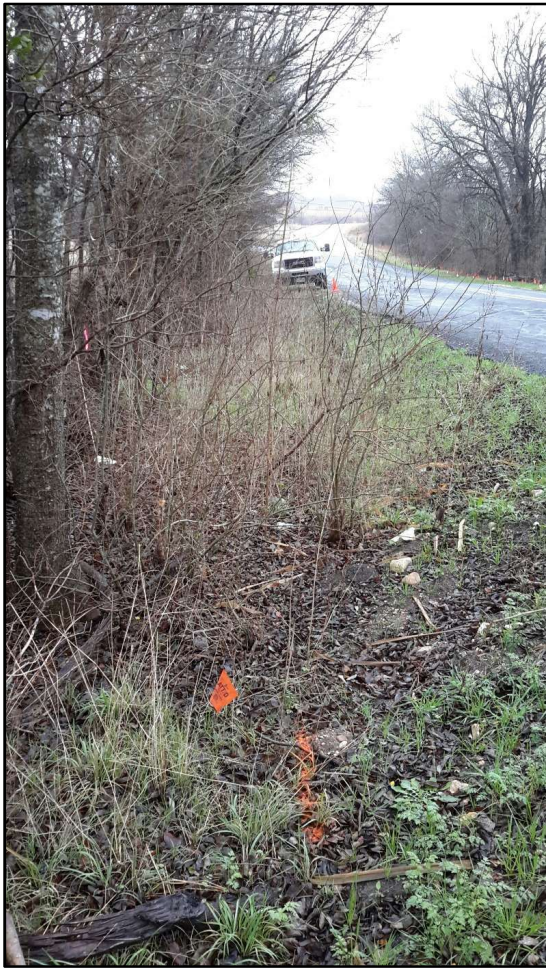
Figure 5. Fill section and marked utilities along eastern side of APE, facing south.
