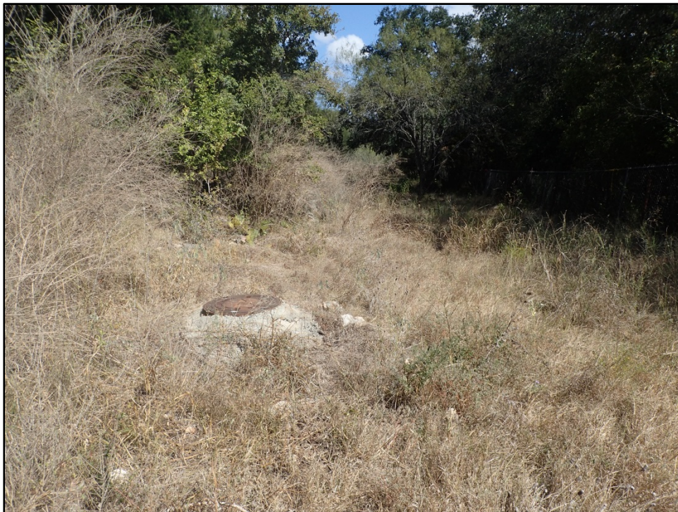
Figure 3: Sanitary sewer line along the project area's southeastern border, facing northeast.
