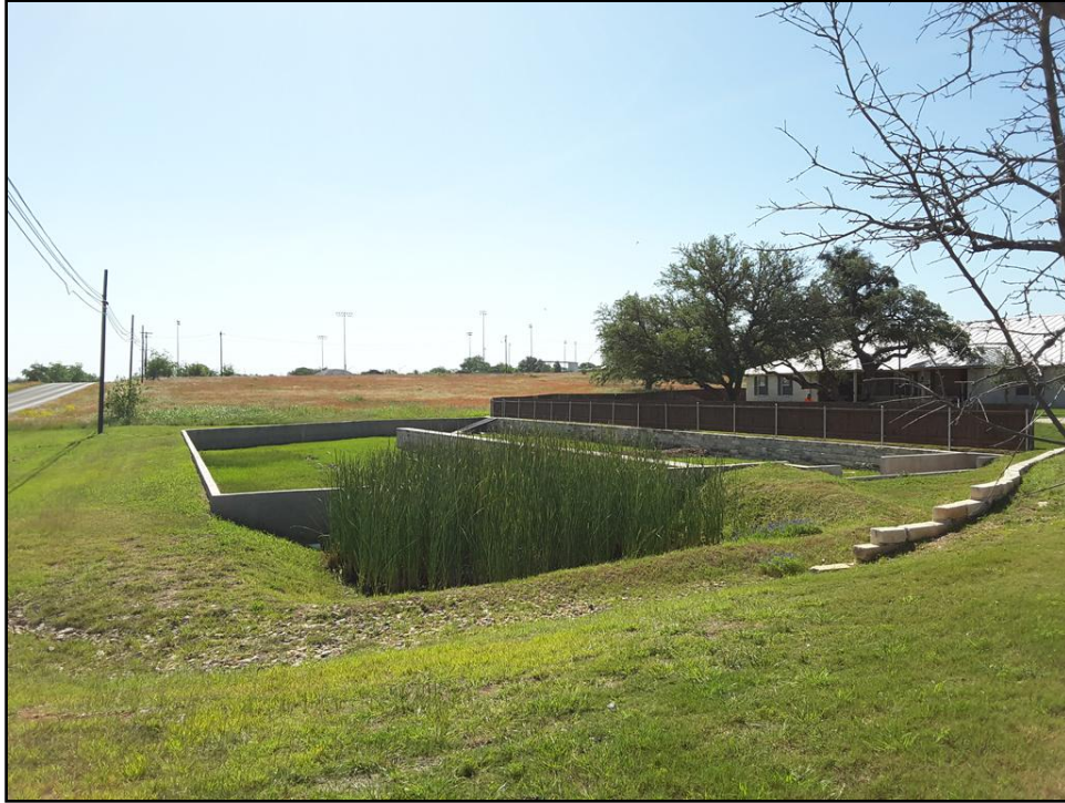
Figure 10. Large cement reservoir next to apartment, view southeast.
