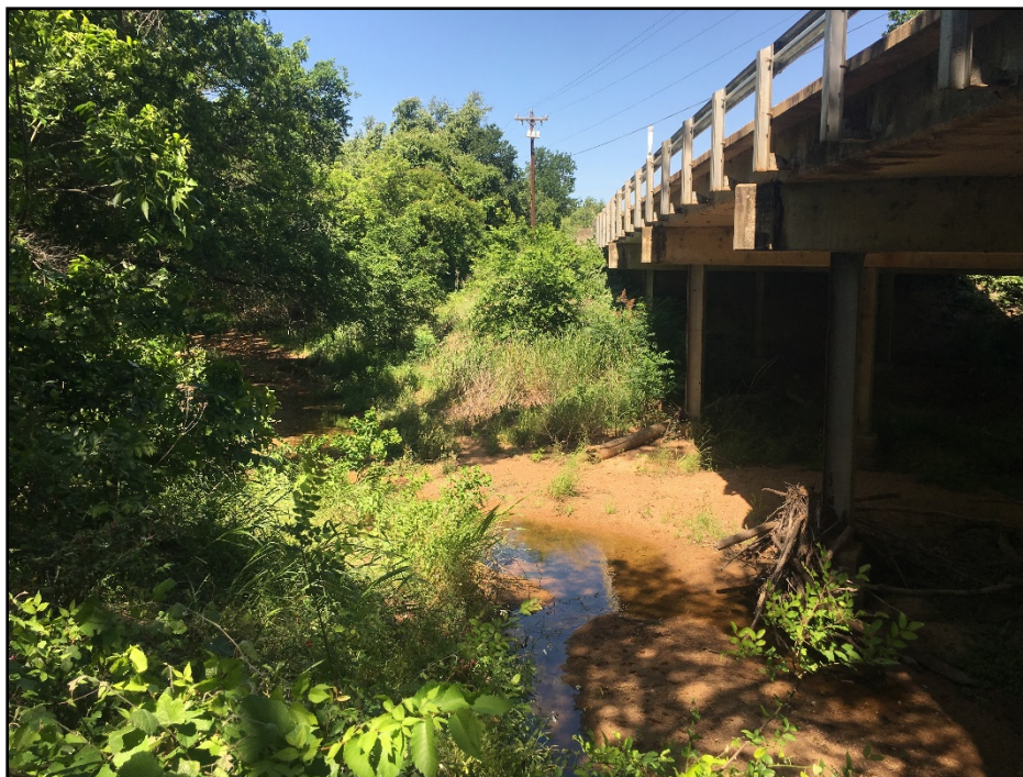
Figure 7. View of the channel of Flag Creek and the adjacent bridge.
