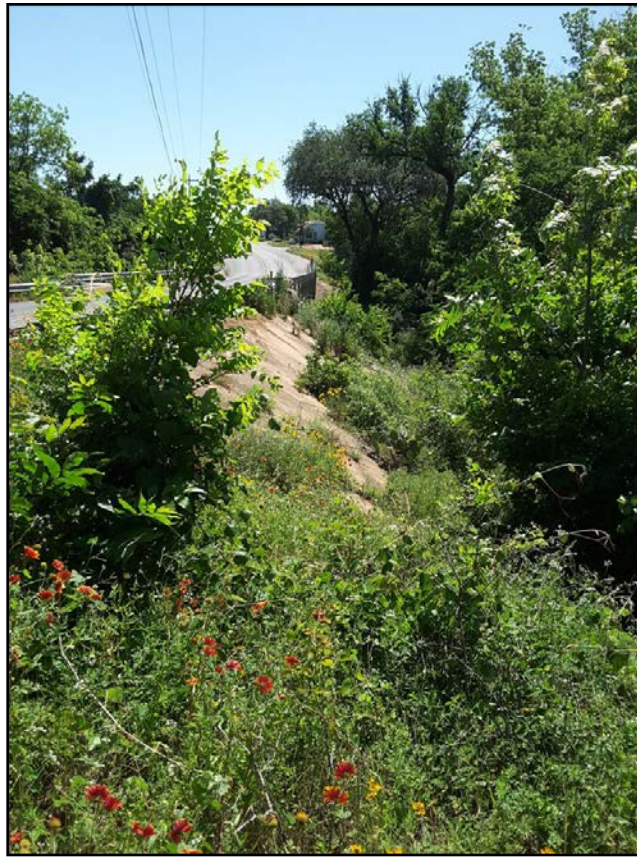
Figure 6. Overview of bridge crossing at Flag Creek, view east.
