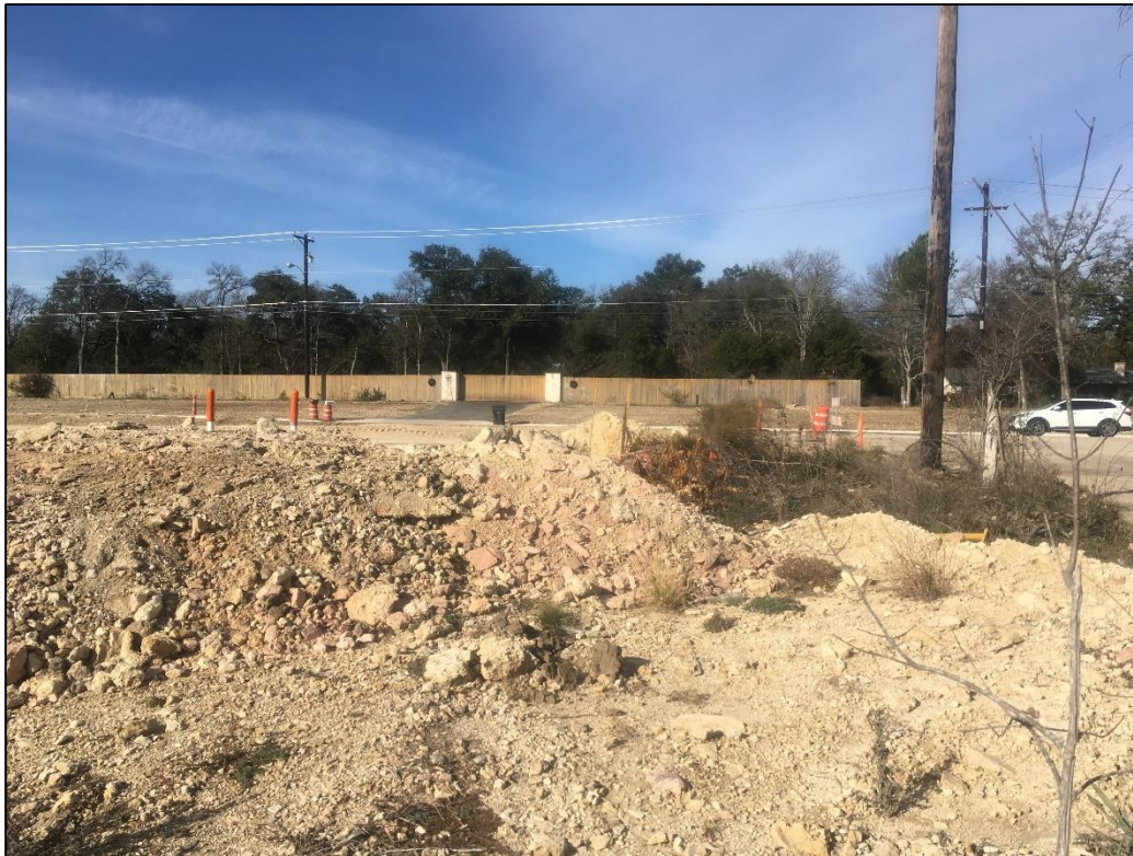
Photo 11. Project APE near 41BL1379. Note disturbances from construction. View to the west.
