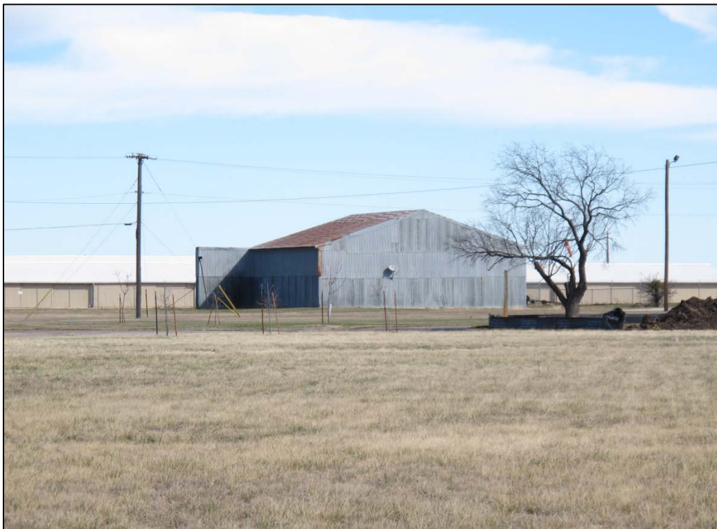
Figure 16. Storage building (Resource 12) visible on 1967 topographic map with warehouses visible on 1957 topographic map (Resources 8-10) in background
