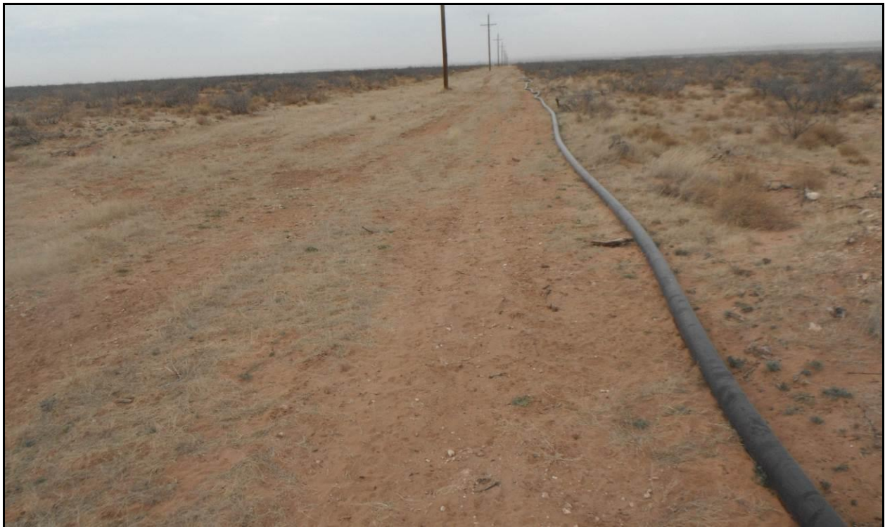
Figure 2-2. View of access road portion of Project Area, facing north
