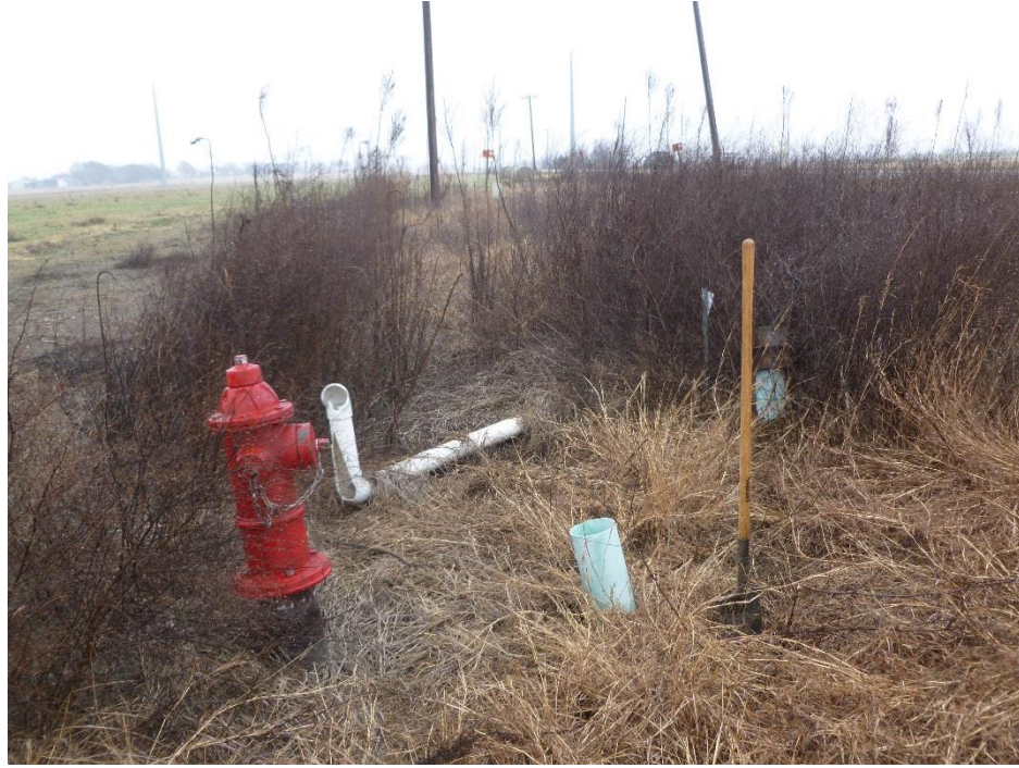
Figure 6. View southeast of multiple utilities and disturbances in vegetated area near intersection of SH 130 and East Pecan Street. Shovel test 3 excavated just off screen at right.
