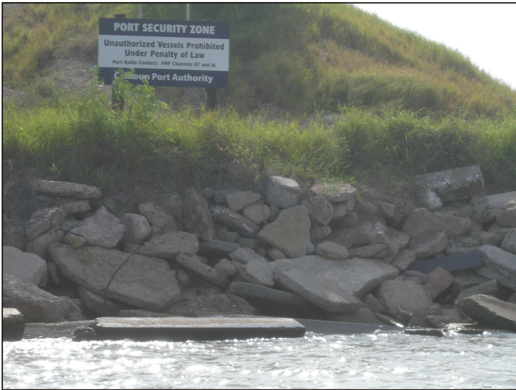
Plate 2. Detail of the concrete and rebar shore line protection material. Note inclusion of metal rebar, a material which will create magnetic anomalies.
