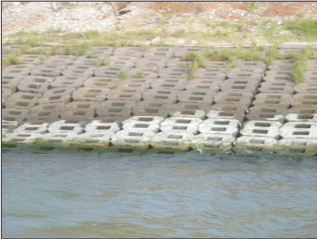
Plate 4. Detail of concrete erosion mats attached by wire cable. The metal in the cable is a source for magnetic anomalies.
