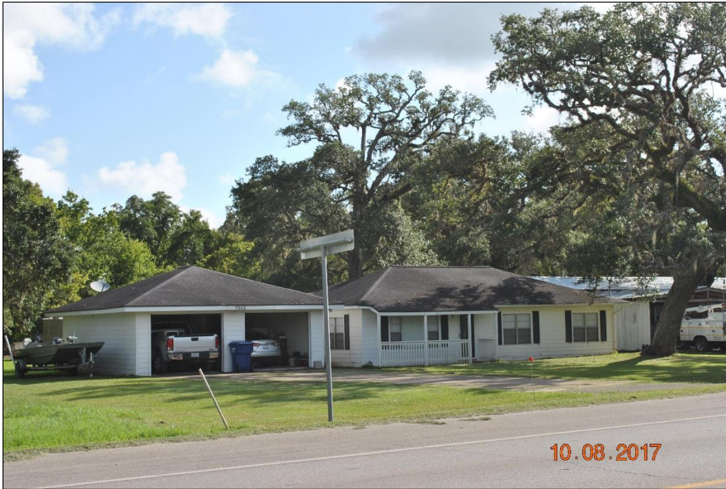
Figure 14. Resource 3—Dwelling at 9363 FM 254 (Formerly 32 FM 524) (Facing Northeast)
