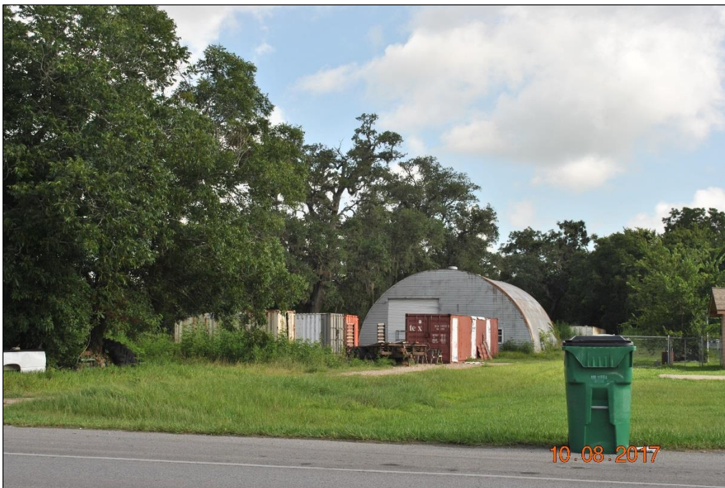
Figure 21. Resource 10—Commercial building 0.2 Mile West of Old Main Street and FM 524 (Facing Northwest)
