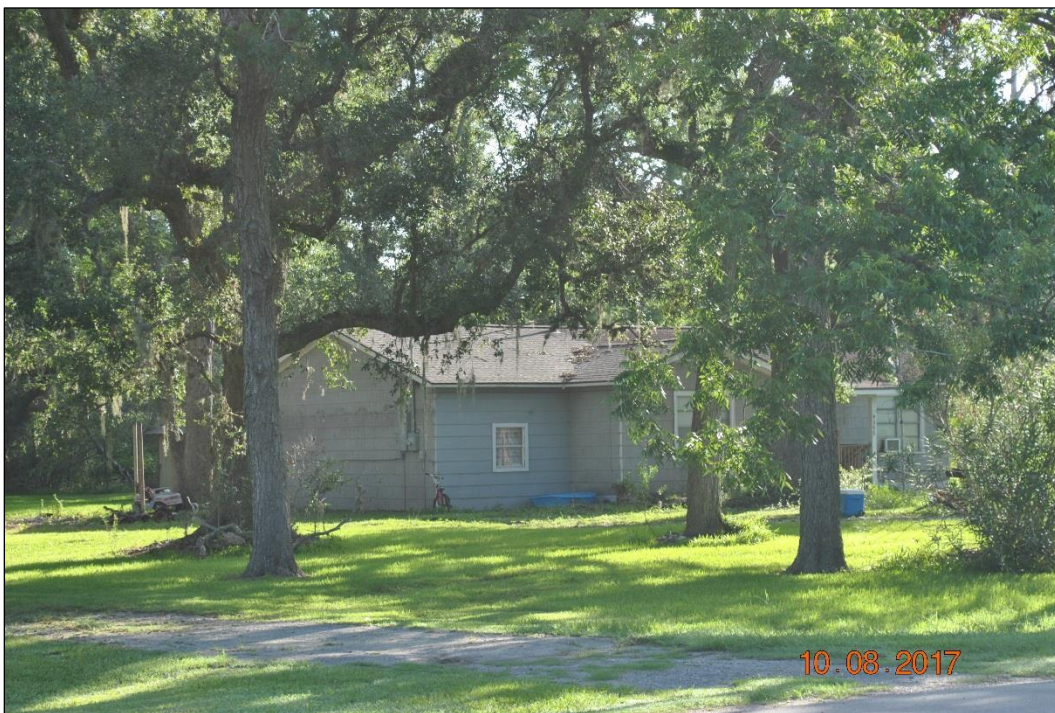
Figure 12. Resource 2—Dwelling at 9355 FM 524 (Formerly 35 FM 524) (Facing Northeast)
