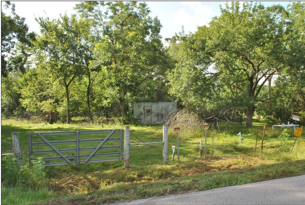
Figure 11. Resource 1—Pipeline Metering Shed on FM 321 (Facing Southeast)
