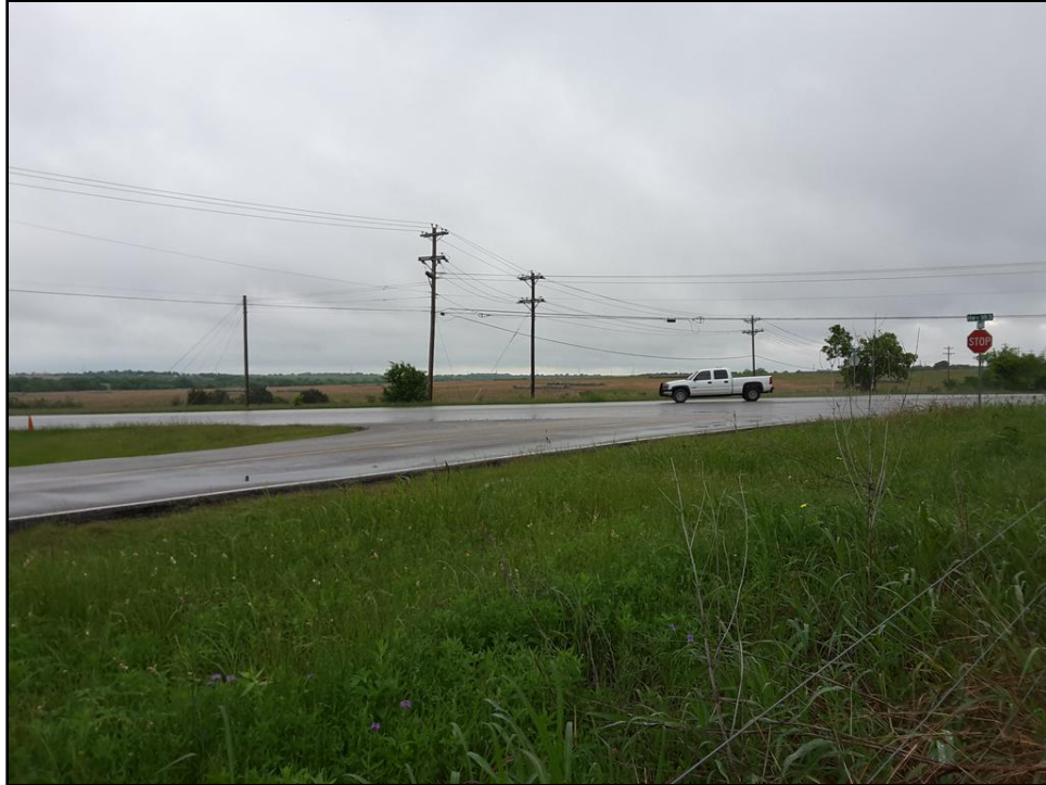
Figure 6. Intersection of US 183 and FM 1625, facing northwest.
