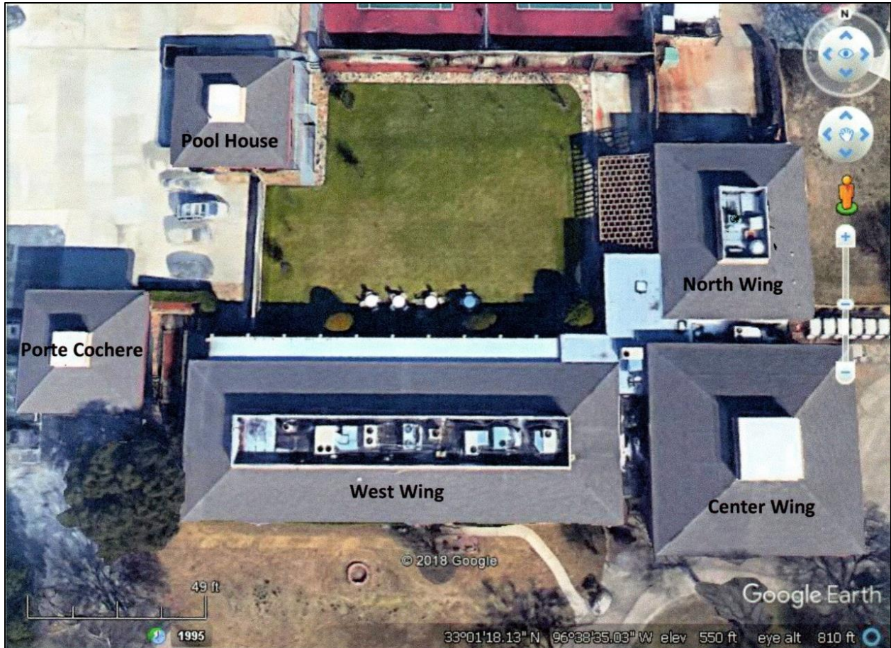
Figure 6. Aerial view of the three wings of the clubhouse, pool house, and porte cochere. Retrieved from Google Earth on February 23, 2018.
