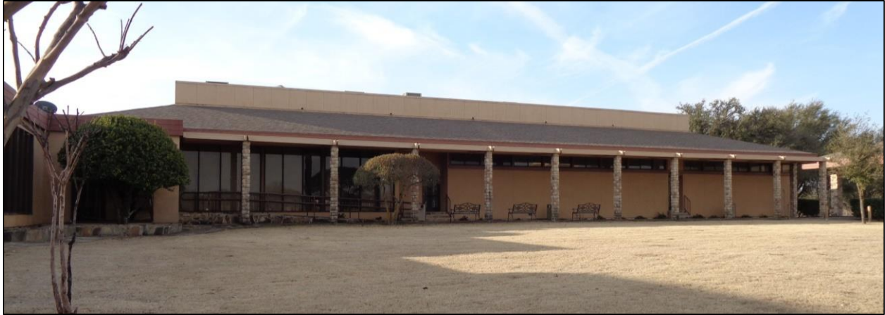
Figure 7. North side of west wing showing canopy. View looking southwest.
