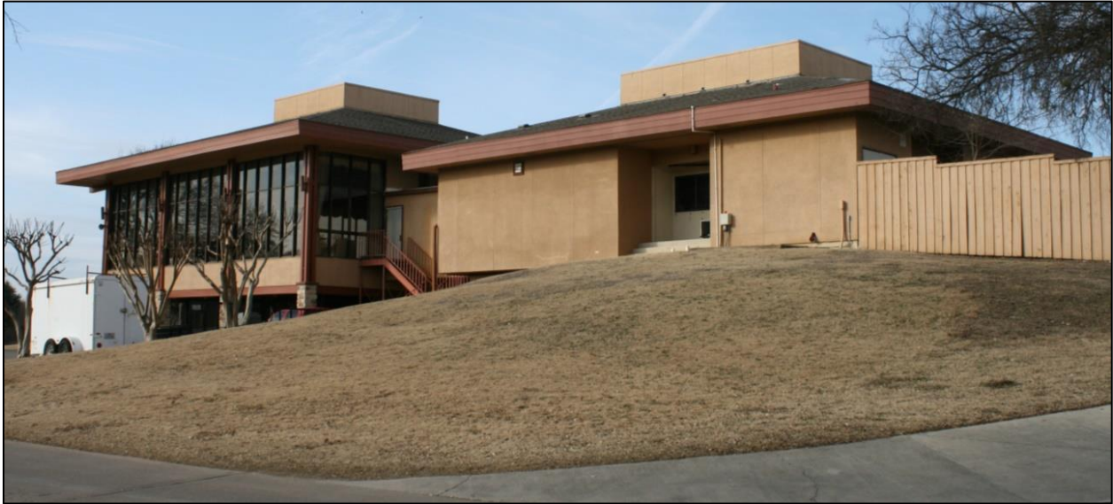
Figure 12. East elevation of center wing and east and north elevations of north wing. View looking southwest.
