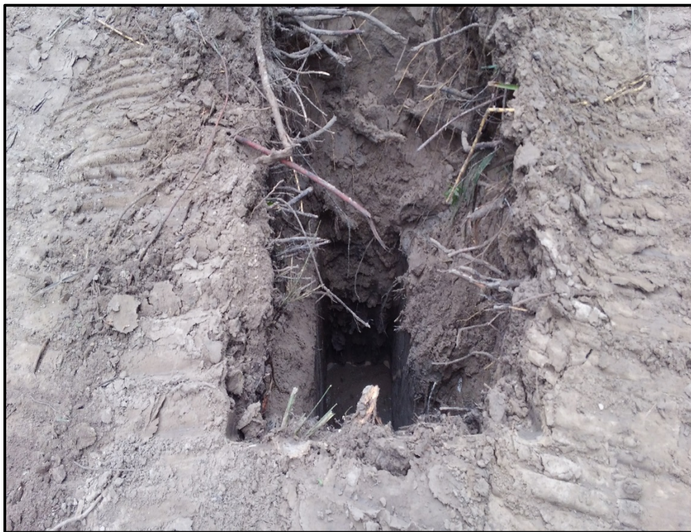
Figure 14. Trench 4 at bottom of project impact.
