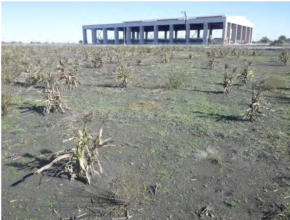
Figure 5. View from APE to EWCEC under construction.
