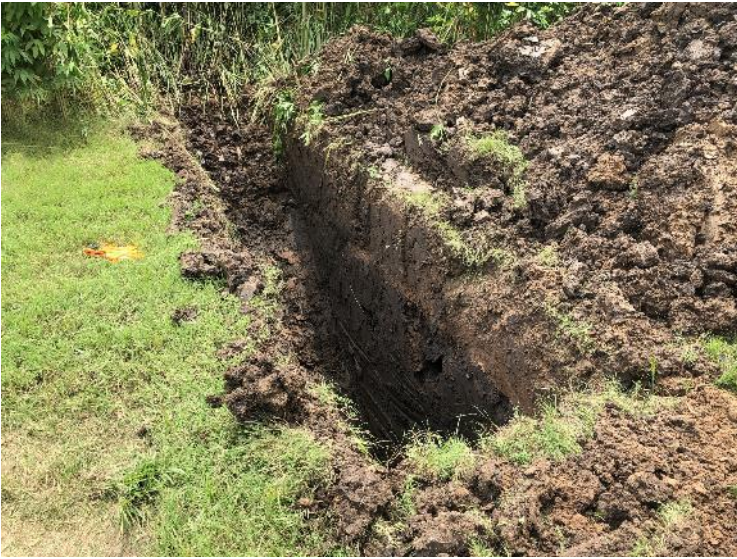
Photograph 15 - Trench 4, view to the southeast.
