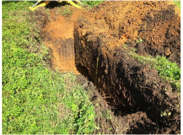
Photograph 10 - Trench 2, view to the west.
