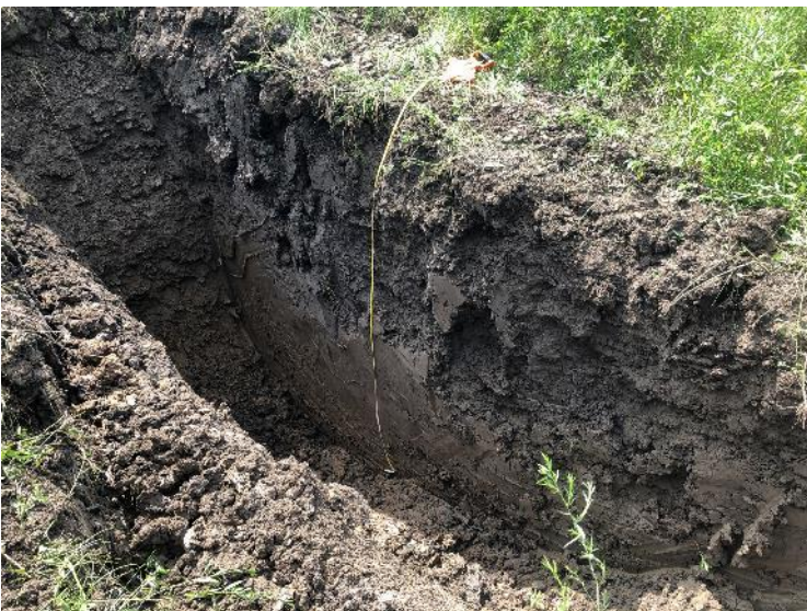
Photograph 11 - Trench 3, view to the southeast.
