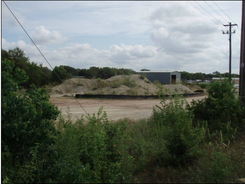
Figure 10. Sand and gravel operation at western end of project area, facing north.
