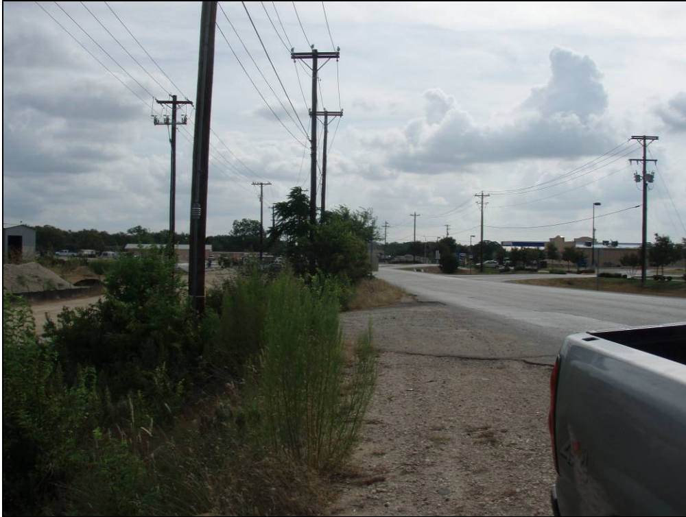
Figure 8. Overhead powerlines which parallel both sides of the roadway, facing east.
