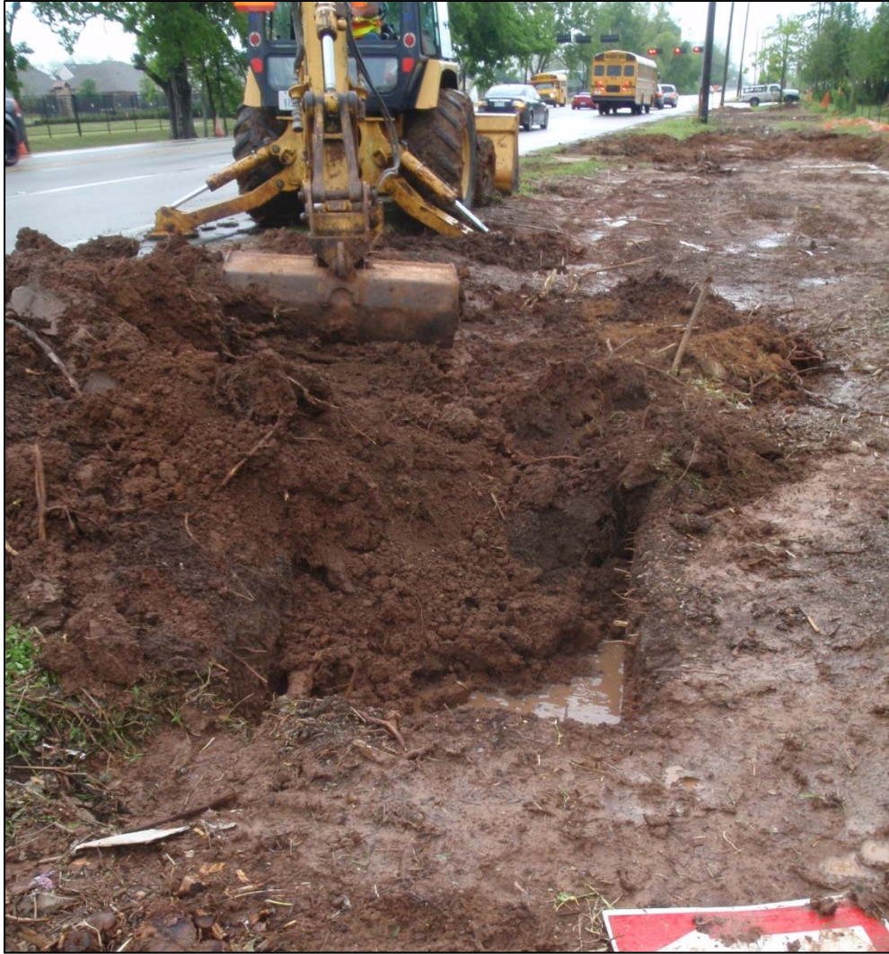
Figure 13: Backfilling of scrape. Note standing water in trench.
