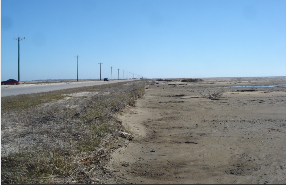
Figure 7: View along SH87 beachfront.
