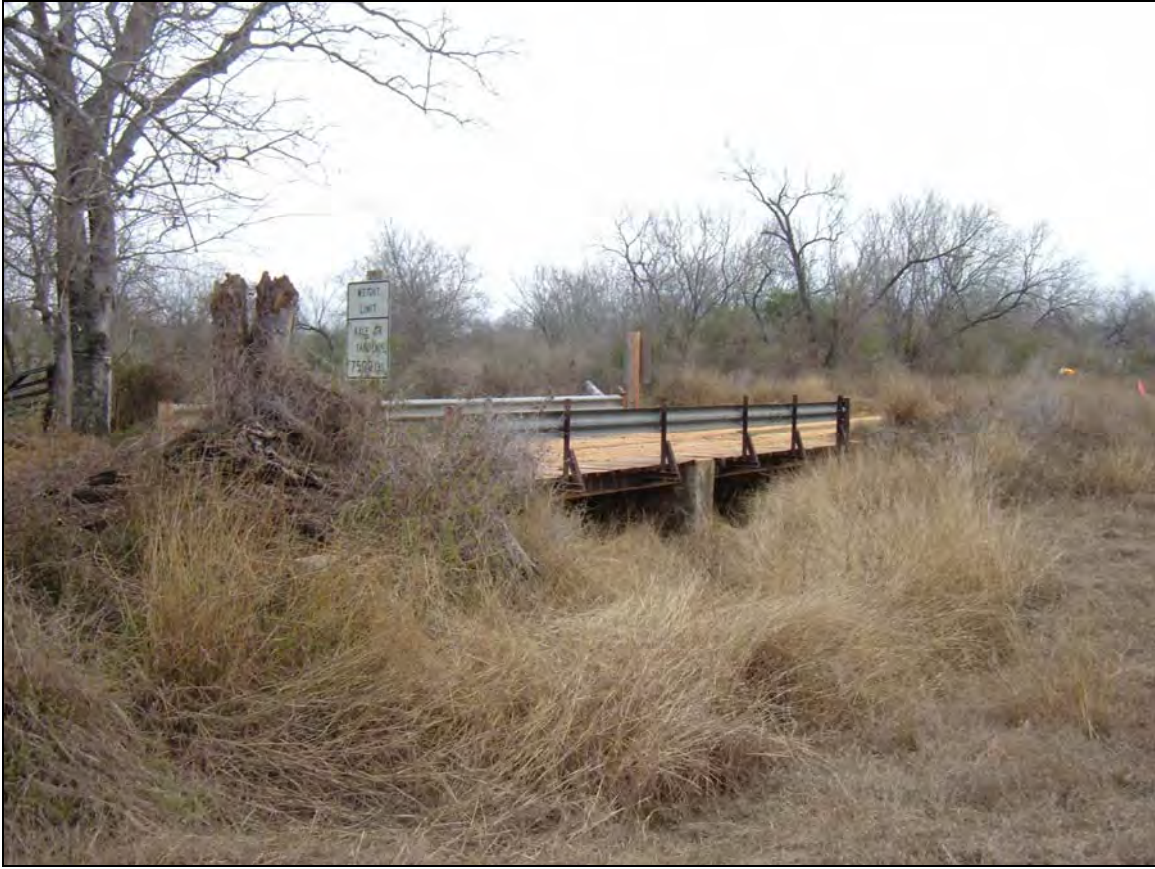
Figure 11. Overview of the Applewhite Lane at Mustang Creek bridge, facing east.
