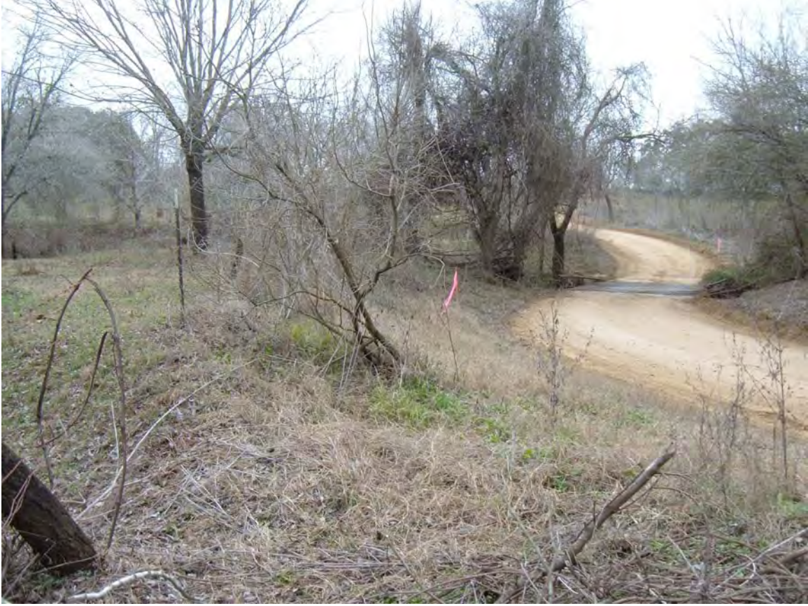
Figure 10. Overview of road cut below grade along eastern approach; facing west.
