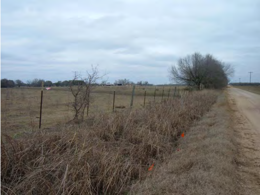
Figure 7. Overview of fence line and buried utility along Byrd Road; facing north.
