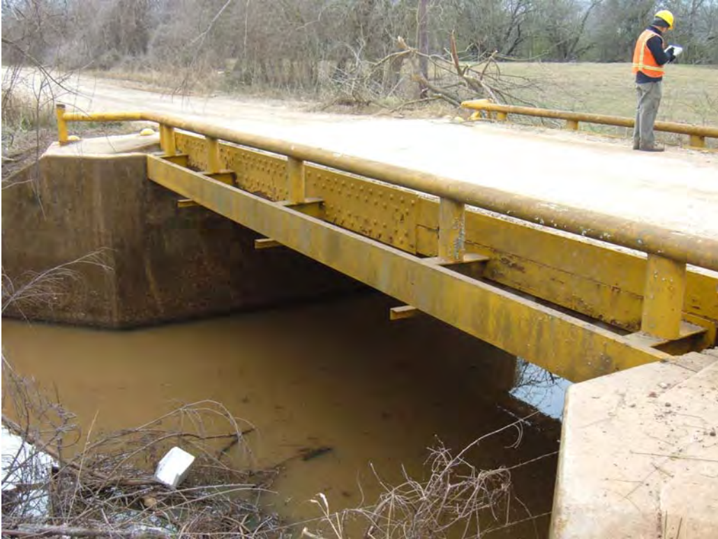
Figure 4. Overview of Byrd Road at Lucas Creek bridge; facing southwest.
