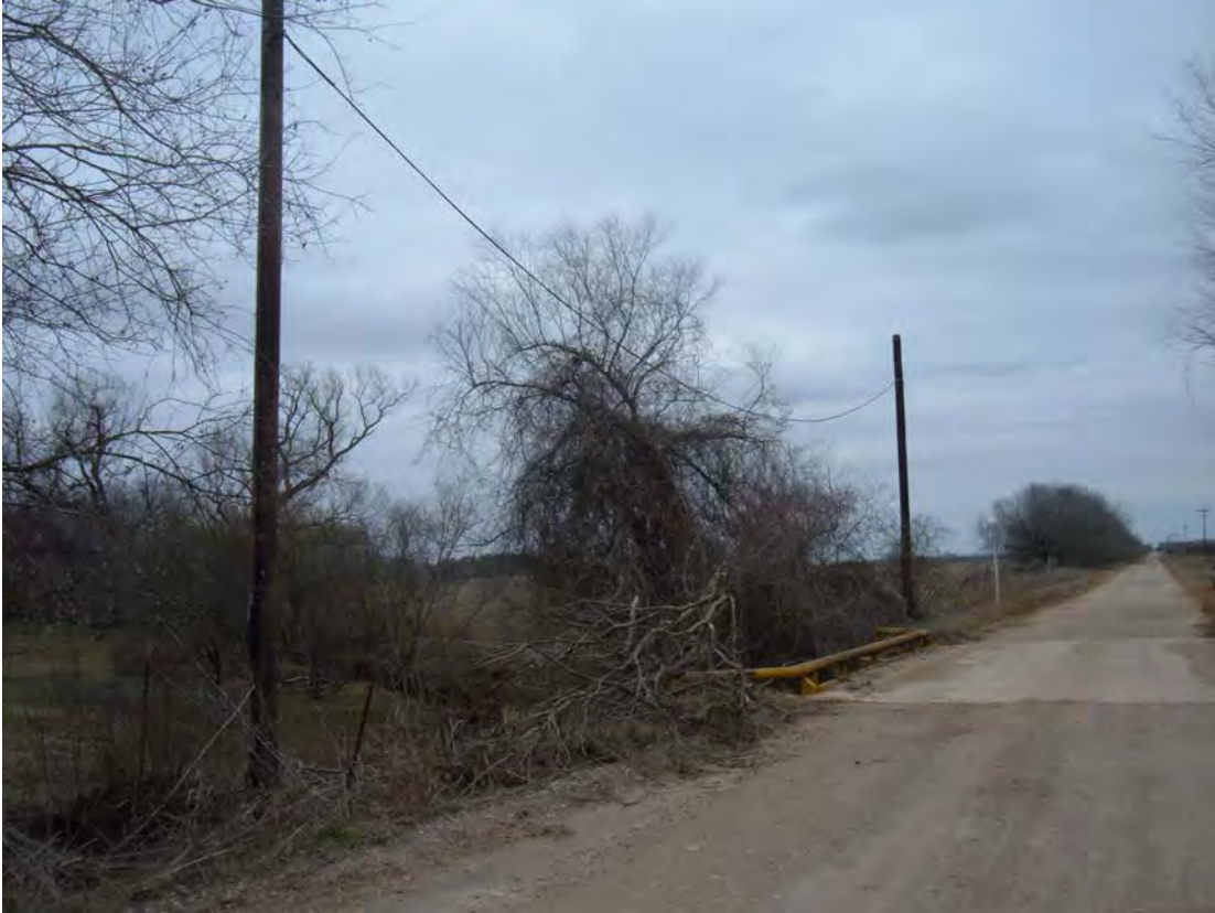
Figure 6. Overview of buried and overhead utility along Byrd Road; facing northwest.
