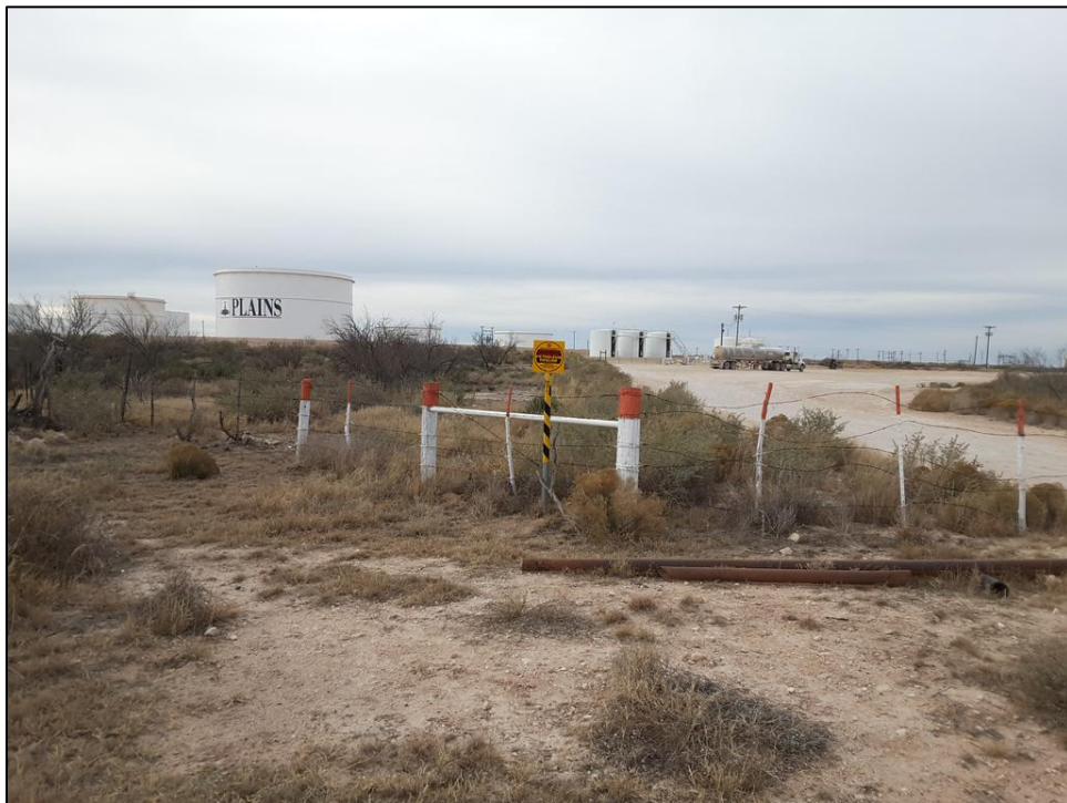
Figure 7. Example of oil-related disturbances and access roads from shovel test MM008, facing south.
