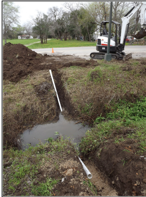
Figure 4-20. View of excavated trench crossing the acequia.
