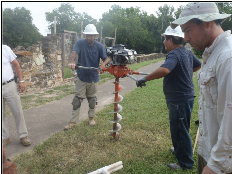
Figure 3-1. Gas powered auger used to excavate bollard and auger holes.
