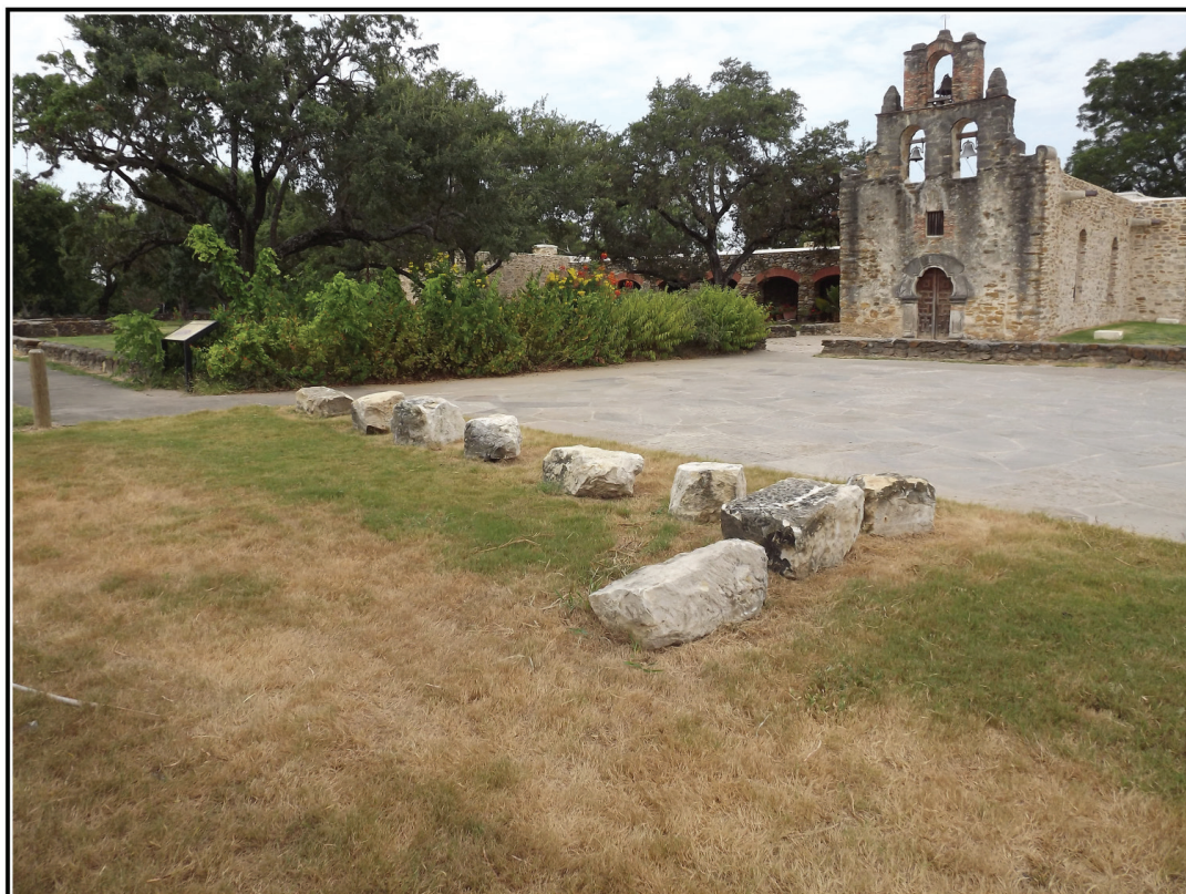
Figure 4-7. Treatment of Feature 1 area (facing southwest).
