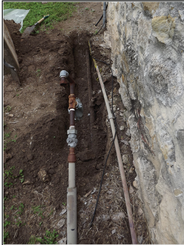
Figure 4-9. Excavation for the water valve box replacement.
