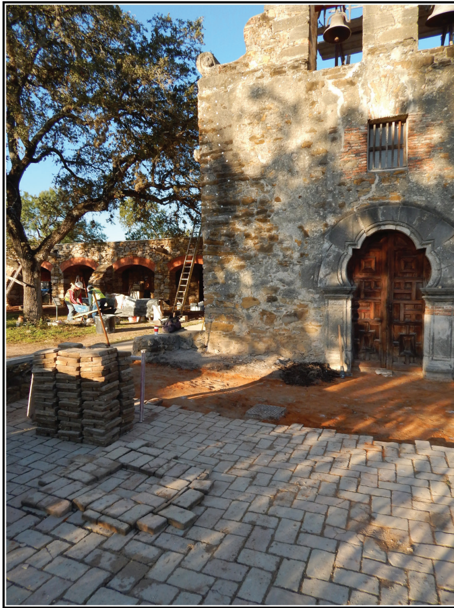
Figure 4-25. The removal of fill underneath pavers in front of the church.
