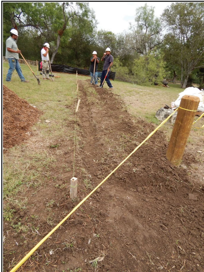
Figure 4-24. Trench excavated for drainage of rainwater collected in parking lot area.
