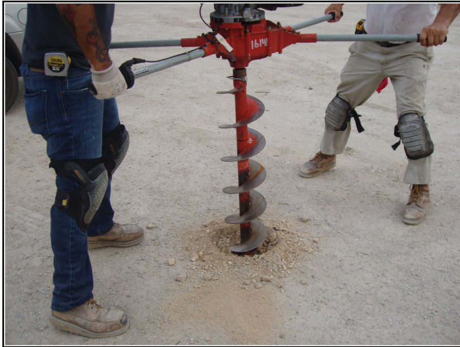
Figure 4-2. Gravel encountered in auger tests.
