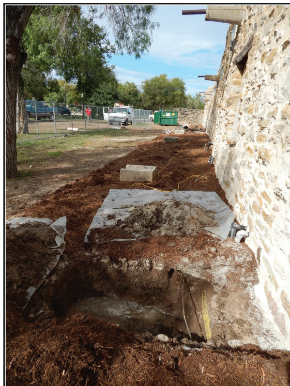
Figure 4-10. Excavations associated with sewage blockage.
