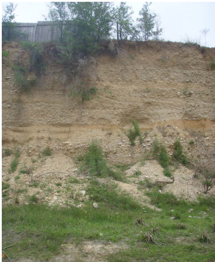
Figure 4: Large piles of loose cobbles and gravels that have eroded out from the south bank wall of Leon Creek, facing southeast
