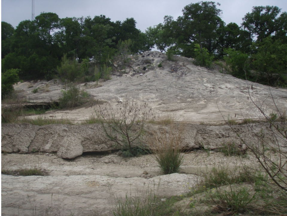
Figure 2: Concrete that has been dumped along the north bank of Leon Creek, facing northwest
