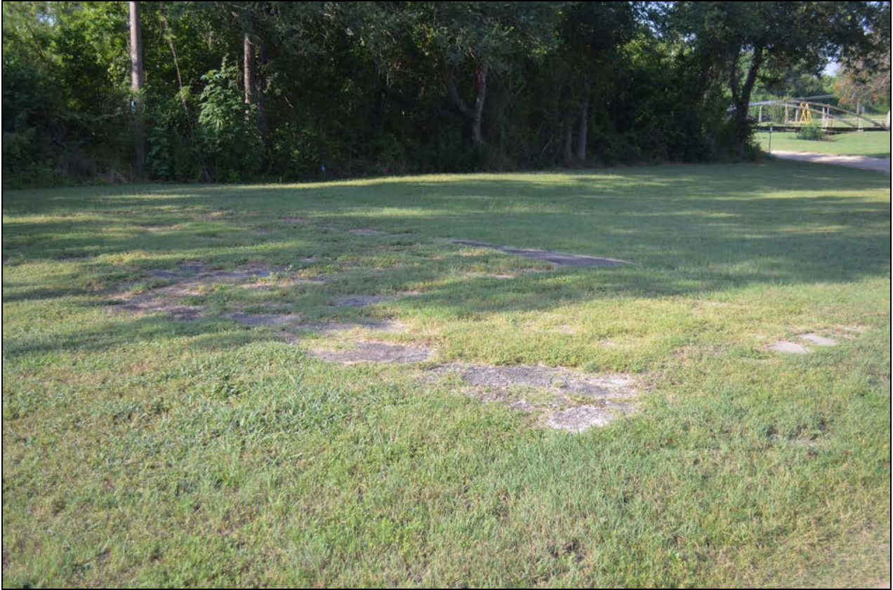
Figure 12. View of cement foundation remnants for the dressing room associated with the former Parkview Pool.
