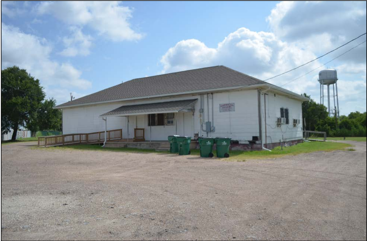
Figure 7. Northeastern view of the American Legion Building/Old Hilltop School.
