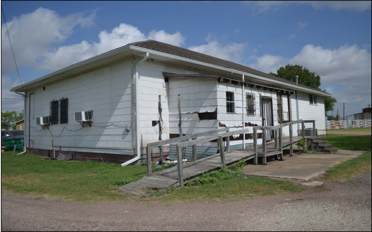
Figure 8. Northwestern view of the American Legion Building/Old Hilltop School.
