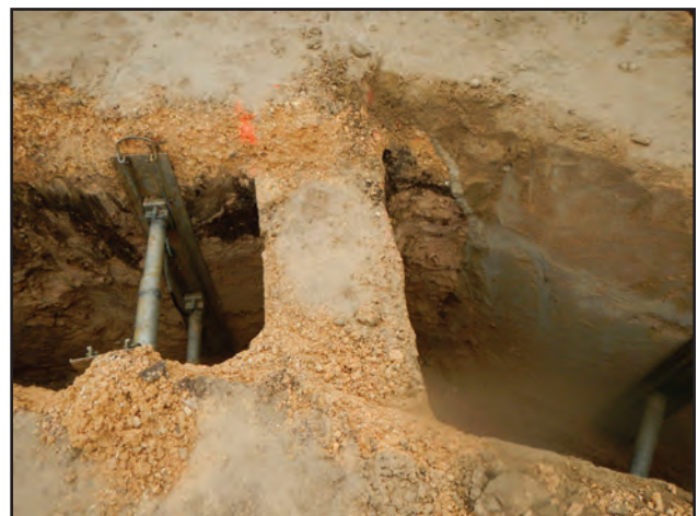
Figure 10.34. Example of existing concrete duct bank utility, facing west.
