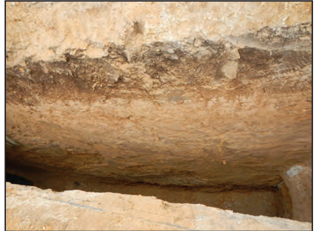
Figure 10.32. Average soil profile for duct bank trench excavations, facing north.
