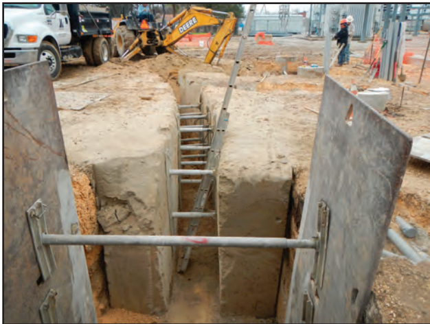
Figure 10.30. West end of duct bank trench excavations, facing east.
