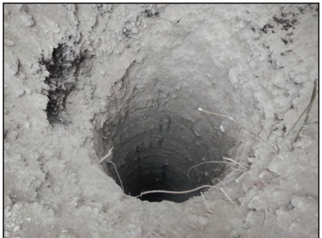
Figure 9.8. Soil profile of pole replacement auger hole, facing west.
