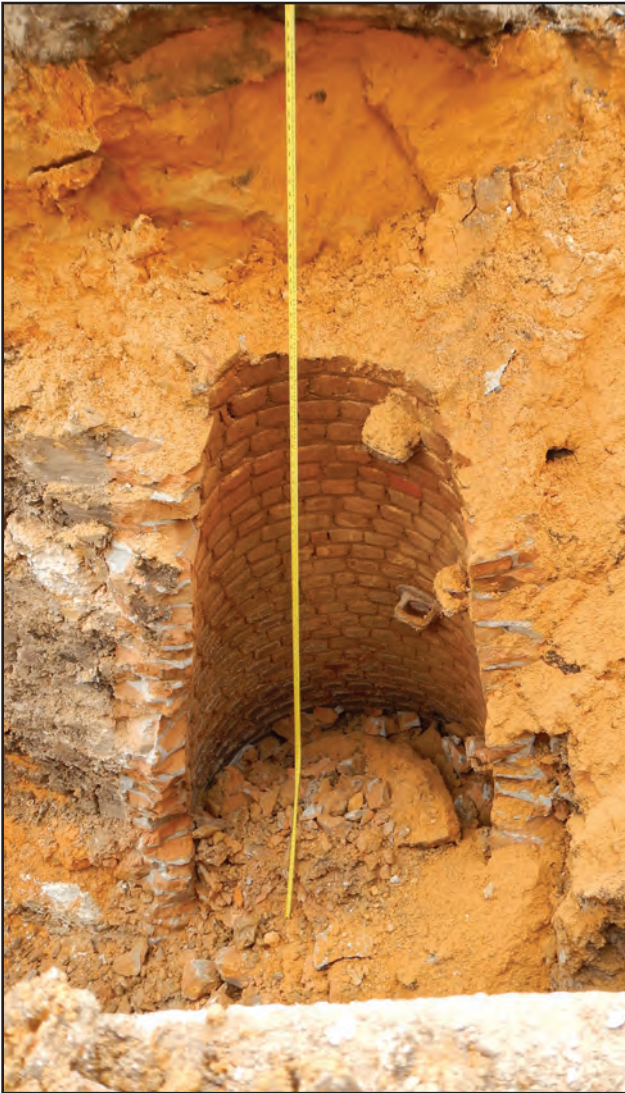
Figure 11.44. Abandoned brick manhole removed from Bore Pit 1, facing south.
