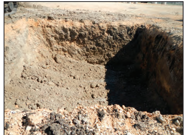
Figure 11.31. Overview of Manhole 11, facing northeast.
