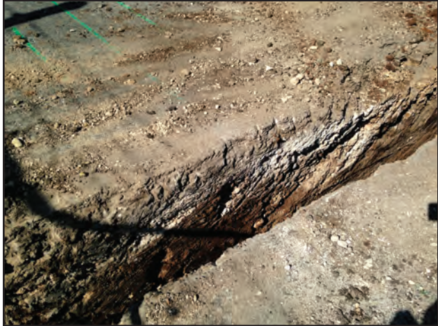
Figure 7.13. East profile of concrete utility bank, facing northwest.
