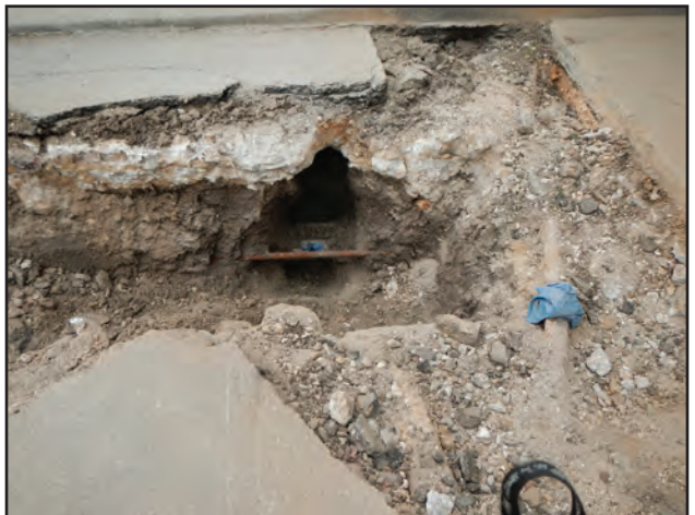
Figure 11.38. Existing utilities within excavations near Manhole 8, facing south.
