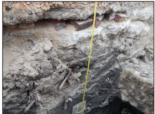
Figure 11.41. Profile view of macadamized red brick layer and wooden timbers near Manhole 4, facing south.
