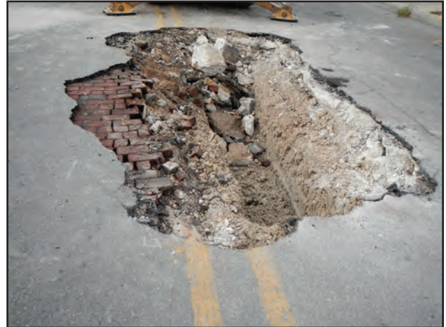
Figure 11.40. Macadamized brick layer near Manhole 8 excavations, facing west.
