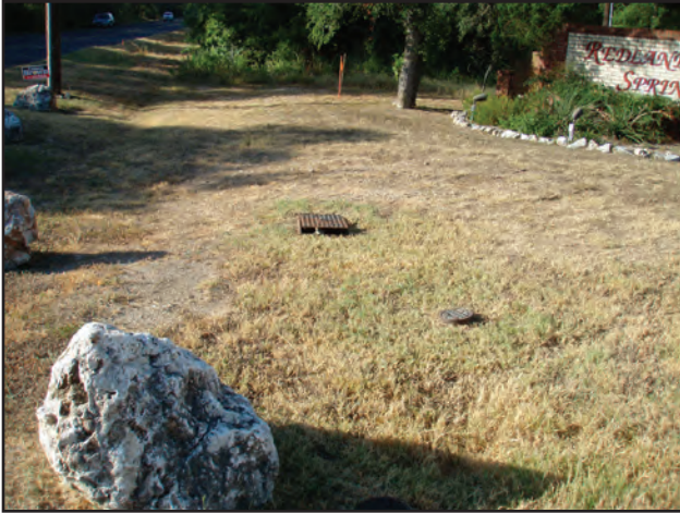
Figure 6.11. Overview of buried utilities within western right-of-way of Bulverde Road, north of Redland Road.
