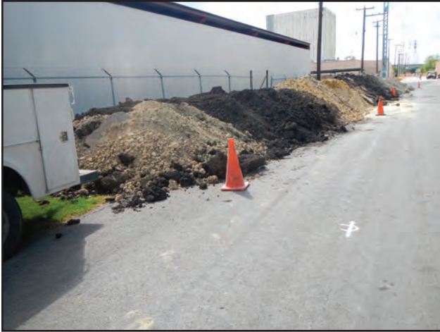
Figure 11.12. Example of relocated spoils from Manhole 1 and 2 excavations, facing southeast.
