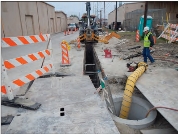
Figure 11.35. Example of trenching excavations associated with manhole; Manhole 4, facing north.
