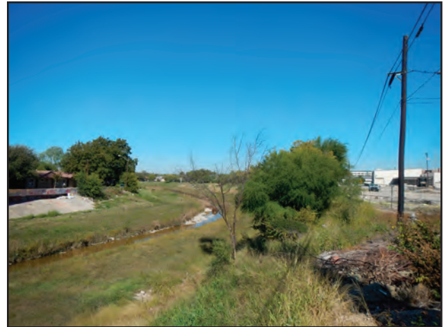
Figure 11.9. Overview of channelized Alazán Creek, facing north-northwest.
