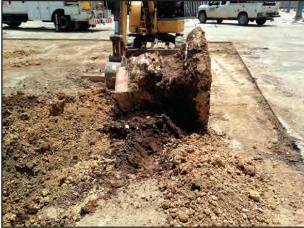
Figure 10.14. Example of extracted pier foundation; Pier 3, facing east.
