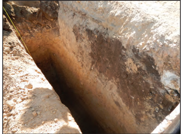
Figure 10.26. Facing southeast, example of manhole profile wall, outer southwest wall, 17 feet in depth.
