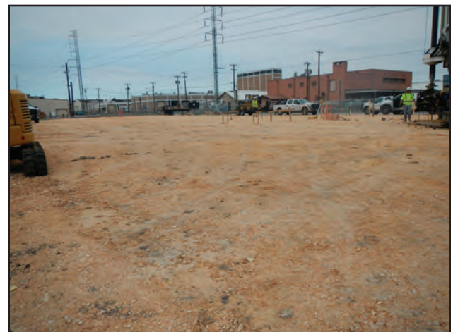
Figure 11.20. Overview of pier foundation excavations, facing northeast.
