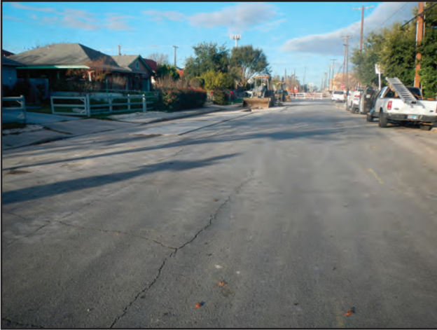
Figure 11.34. General setting overview of the eastern half of Phase 2, facing west.
