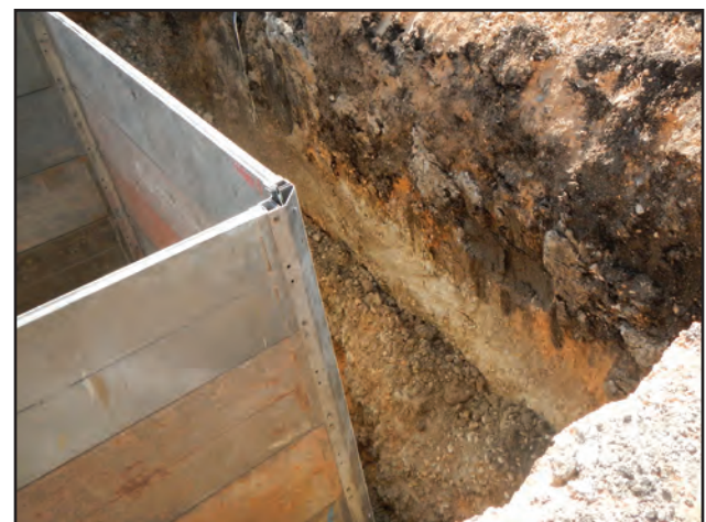
Figure 11.32. Soil profile of Manhole 11, facing southeast.
