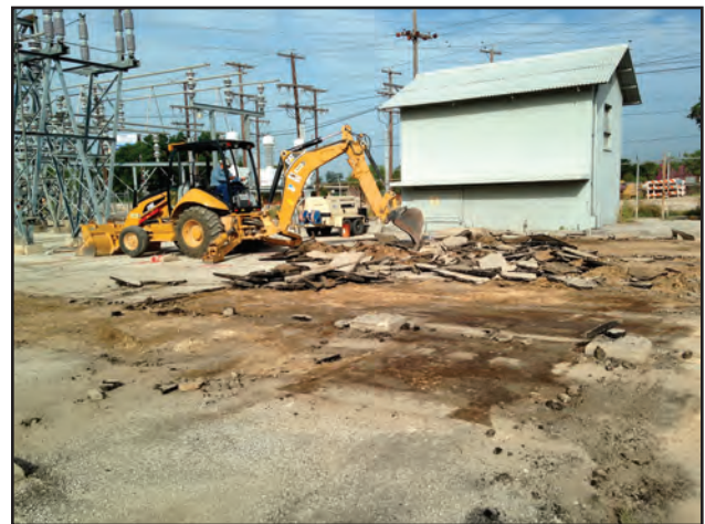
Figure 10.13. Asphalt removal from pier foundation removal area, facing southwest.
