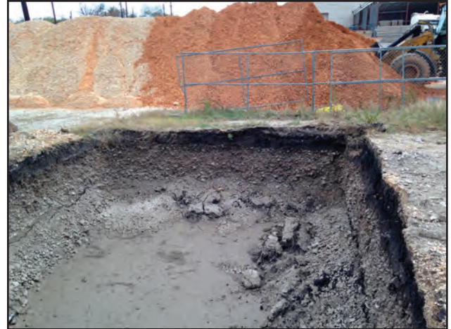
Figure 11.18. Storm Drainage 1 excavation, facing north.
