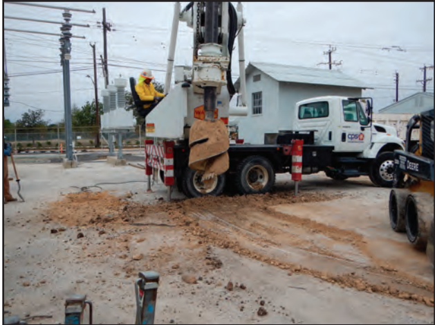
Figure 10.20. Overview of auger excavation process, facing northwest.
