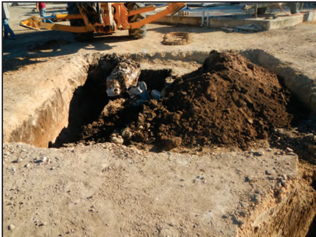
Figure 10.24. Facing northeast, existing utility within manhole excavations, 13.9 feet wide.
