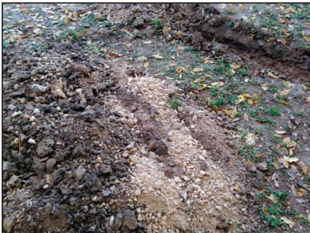
Figure 7.9. Spoil piles from trenching excavation.
