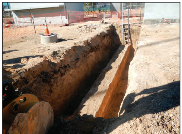
Figure 10.28. Excavation overview of existing utility containing asbestos pipes, facing west-southwest
