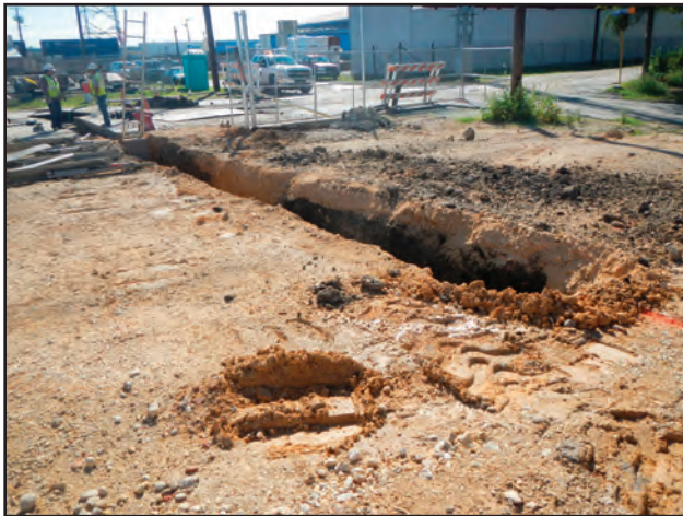
Figure 11.13. Overview of Trench 8 and Manhole 2, facing southeast.
