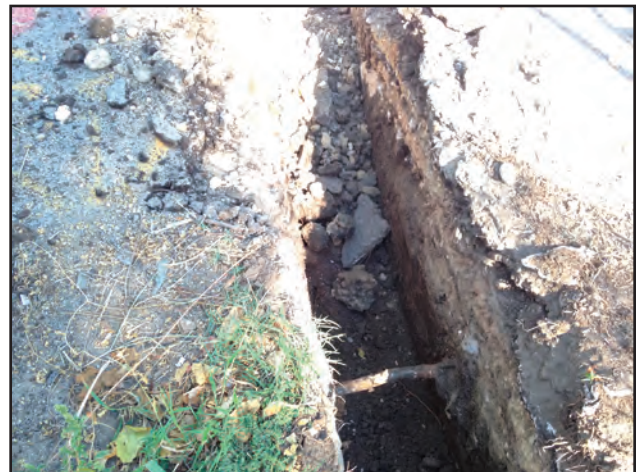
Figure 7.12. Existing waterline at south end of Huizar Road right-of-way, facing north-northeast.
