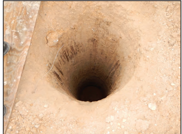
Figure 10.21. Average soil profile for pier foundation replacement excavations, Auger Hole 79.
