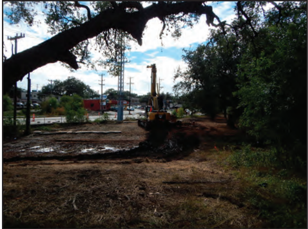
Figure 8.5. Ground disturbance and existing utilities, facing southwest.
