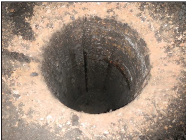
Figure 11.22. Example of soil profile in northern half of substation; Pier 35.
