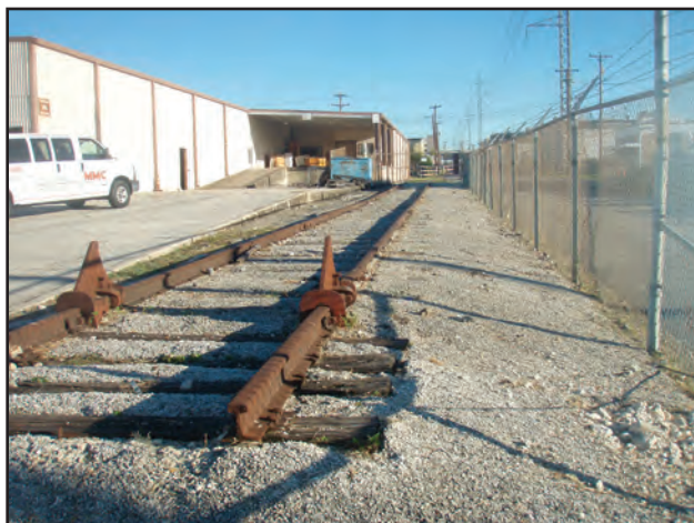
Figure 11.17. Existing rail spur located to the north of the project area, facing north.
