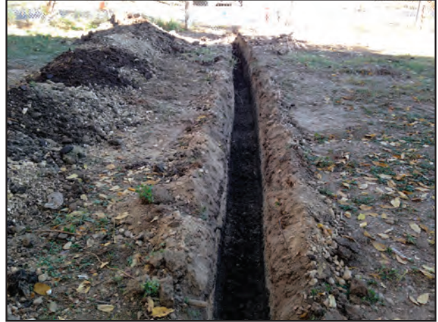
Figure 7.10. Portion of excavations within property boundary, facing north.
