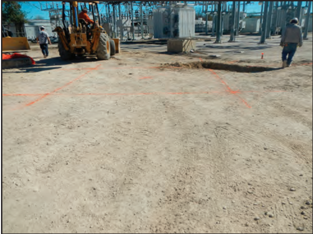
Figure 10.23. Overview of manhole location, facing southeast.
