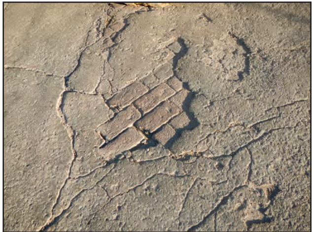
Figure 12.10. Macadamized brick observed on the ground surface next to Tower 2.
