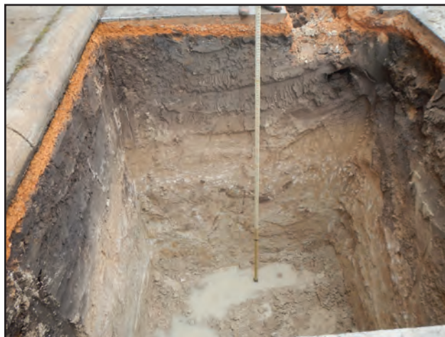
Figure 11.36. Average soil profile of Manholes 3–5 and 9; Manhole 5, facing east.
