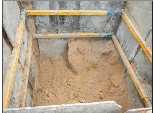
Figure 10.27. Excavated manhole with shoring plates and bracings, facing east.
