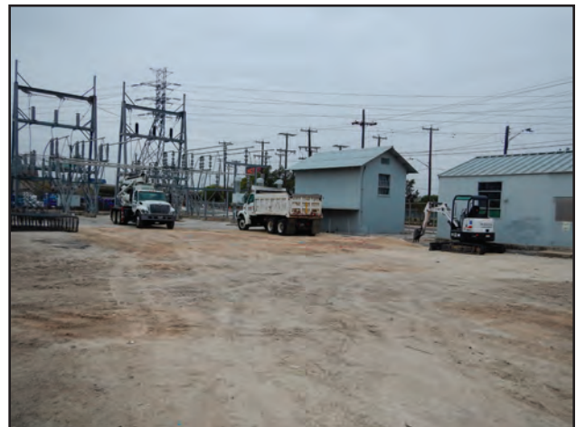
Figure 10.19. Overview of pier foundation removal/excavation work area, facing southwest.
