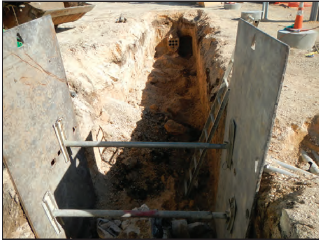
Figure 10.29. Removed existing asbestos utility, facing east.
