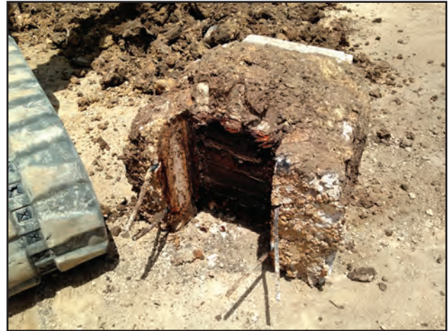
Figure 10.17. Wooden planks beneath Pier 2 foundation, facing south.
