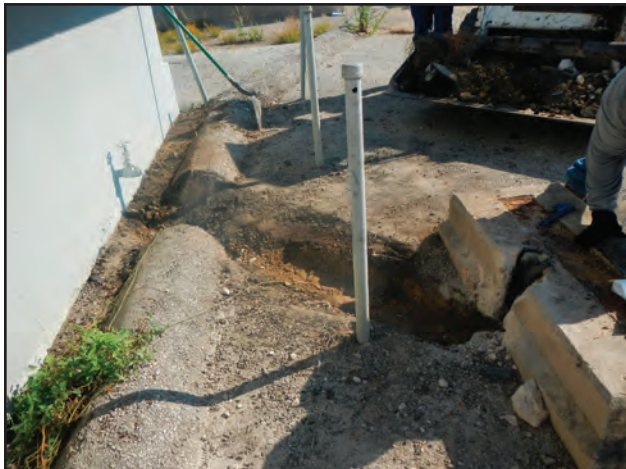
Figure 10.36. Overview of removed Oil House pipe and valve trench, facing north.
