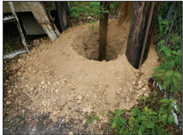
Figure 9.7. Example of spoil deposits around excavation opening, facing west.
