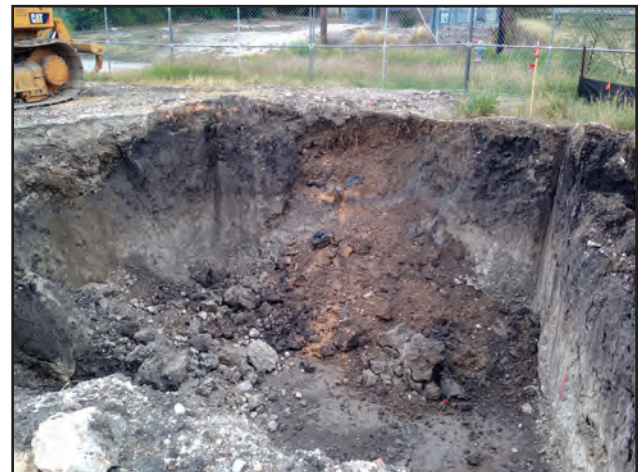
Figure 11.19. Storm Drainage 2 excavation, facing south.
