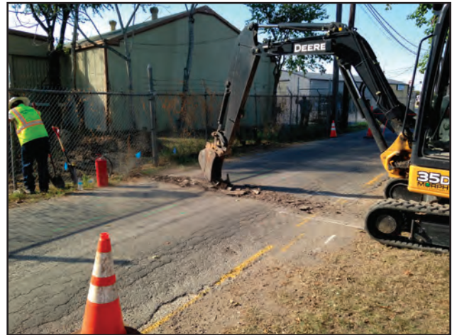
Figure 7.11. Excavations within right-of-way of Huizar Road, facing south-southwest.
