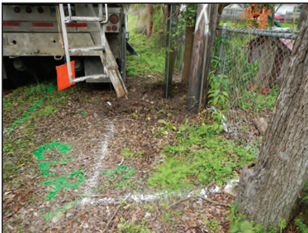
Figure 9.6. Close up of pole replacement location, facing west.
