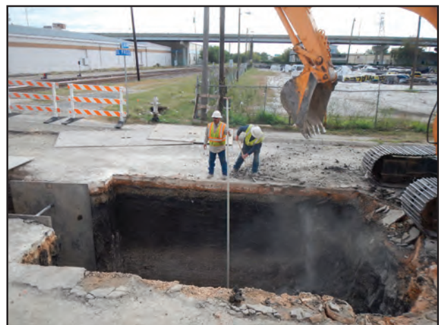
Figure 11.42. Bore Pit 1 excavations, facing south.
