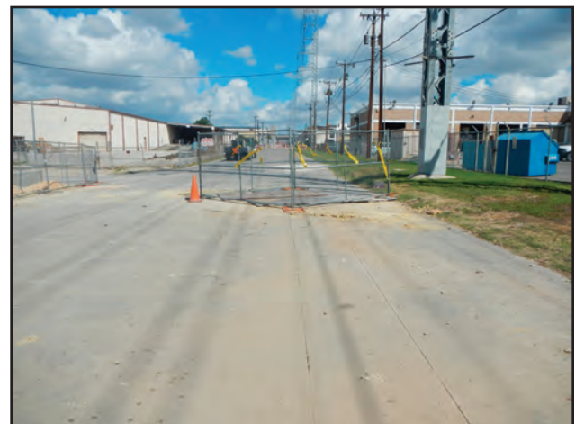
Figure 11.11. Overview of Manhole 1 location, facing north.
