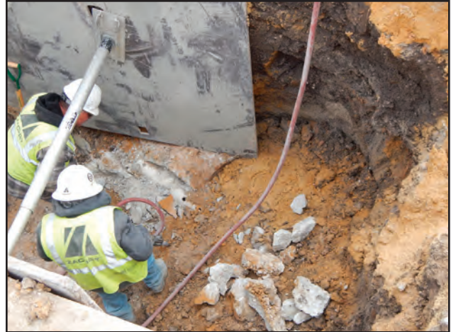
Figure 11.45. Existing PVC pipe at base of brick manhole.
