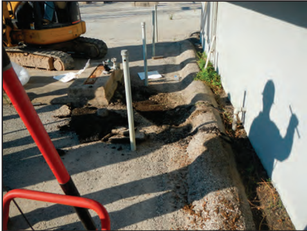
Figure 10.35. Overview of existing Oil House pipe and valve removal, facing south.
