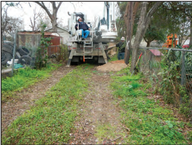
Figure 9.5. Pole replacement location within alleyway, facing west.
