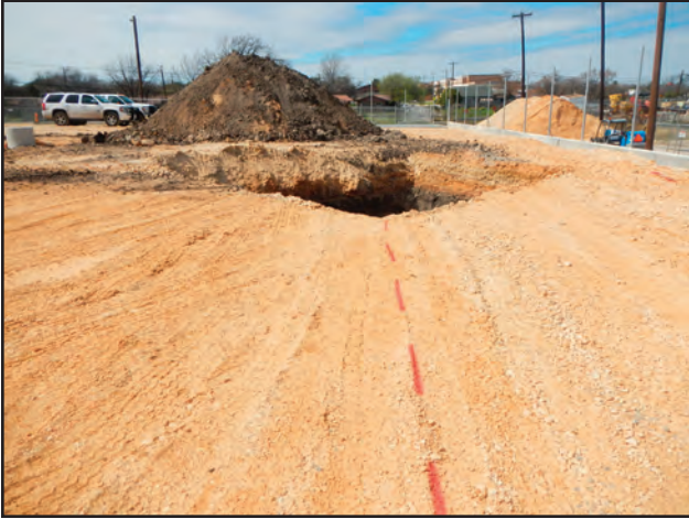
Figure 11.27. Overview of Manhole 10, facing west.
