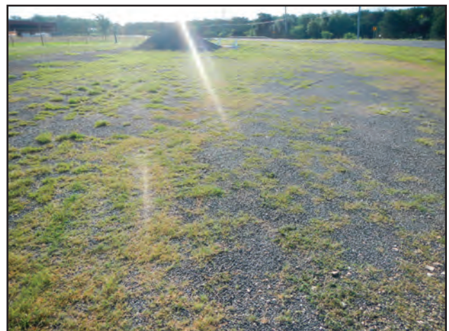
Figure 5.10. Example of asphalt and gravel patches, facing east.
