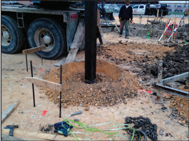
Figure 11.21. Example of pier excavation process; Pier 12, facing northeast.
