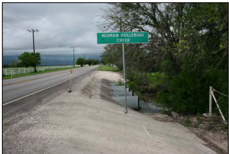
Figure 4. Overview of existing structure at Woman Hollering Creek; facing north.
