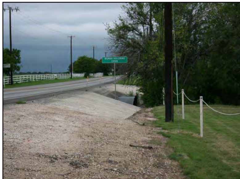
Figure 6. Overview of concrete and gravel apron along east side of roadway; facing north.
