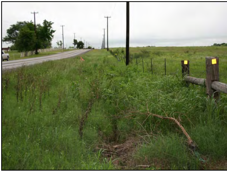
Figure 3. Rolling topography along south approach of project area; facing south.
