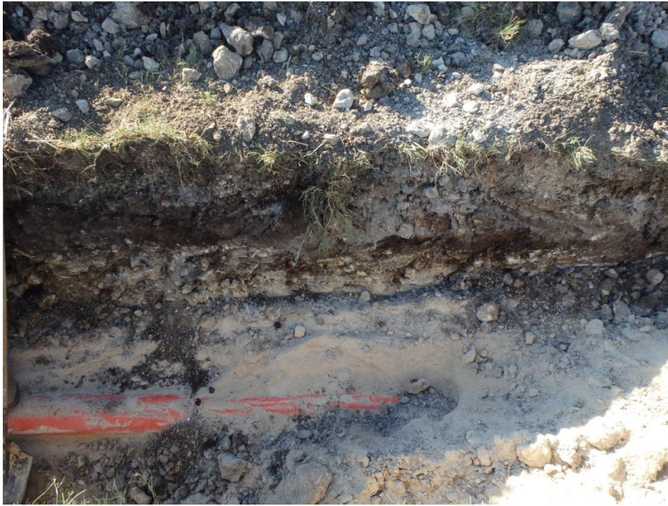
Figure 4-5: Location 3 Profile, Facing South (Existing Telecommunication Line in Foreground)
