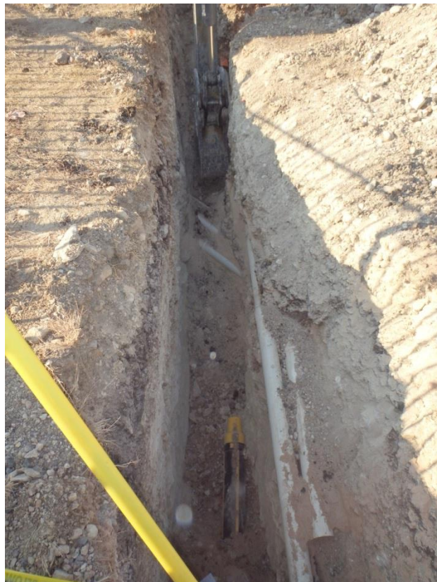
Figure 4-7: View of Buried Telecommunication Lines (Project ROW, Location 4)
