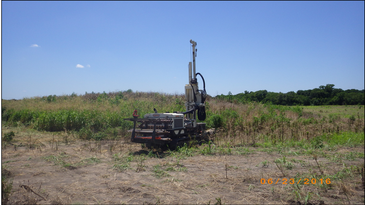
Figure 9. The dirt mound west of the old channel, as seen looking southeast. The machinery in the foreground is a boring rig being used by environmental scientists working at the development site.
