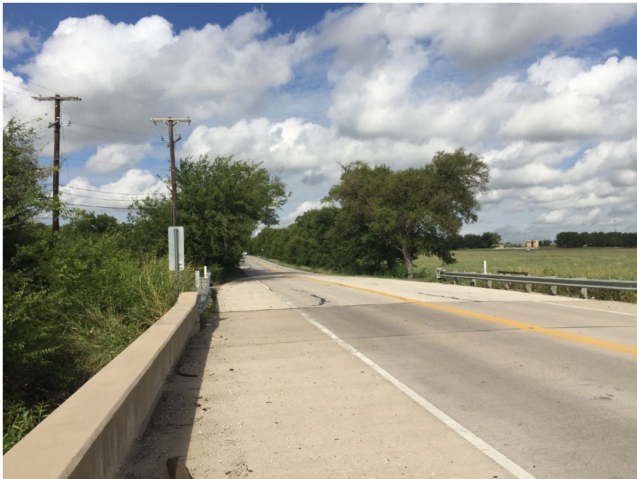
Photo 4. Overview of APE crossing Avondale Haslet Road, facing west
