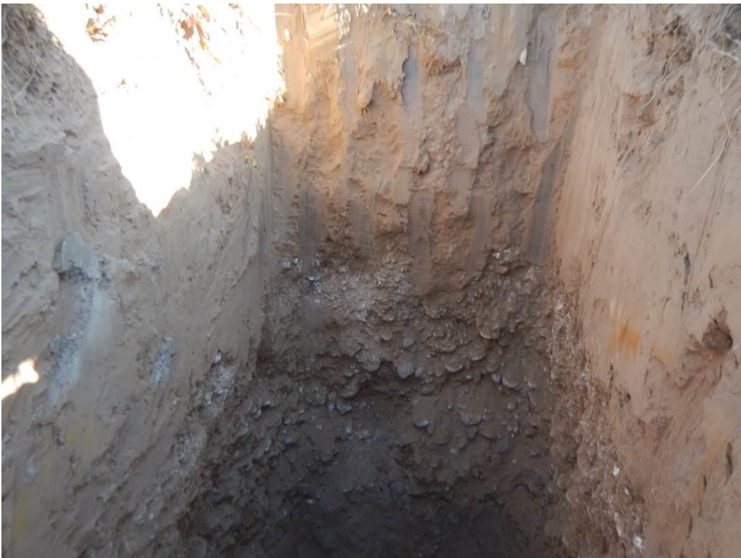
Figure 18. Profile of a typical trench (BH1) with deeply buried road gravels.
