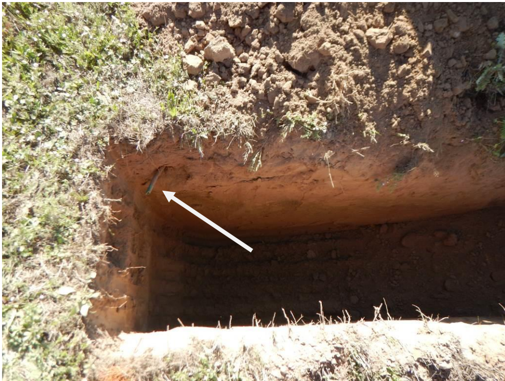
Figure 14. Buried PVC pipe within backhoe trench #4 (BH4)
