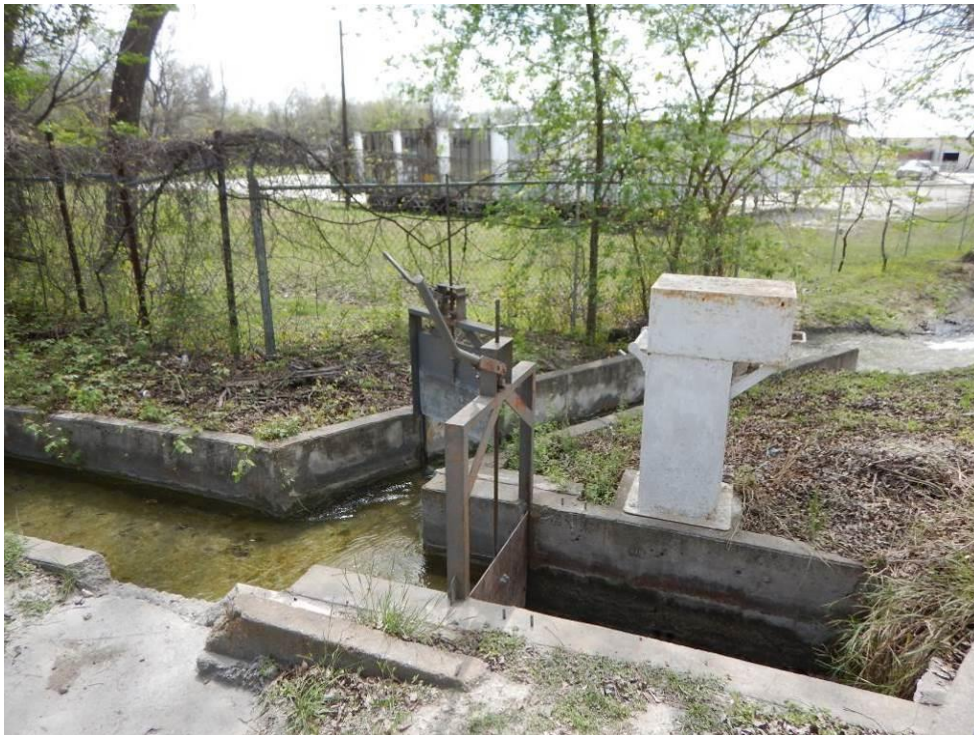
Figure 11. Historical irrigation structures adjacent to the project APE, facing northeast.
