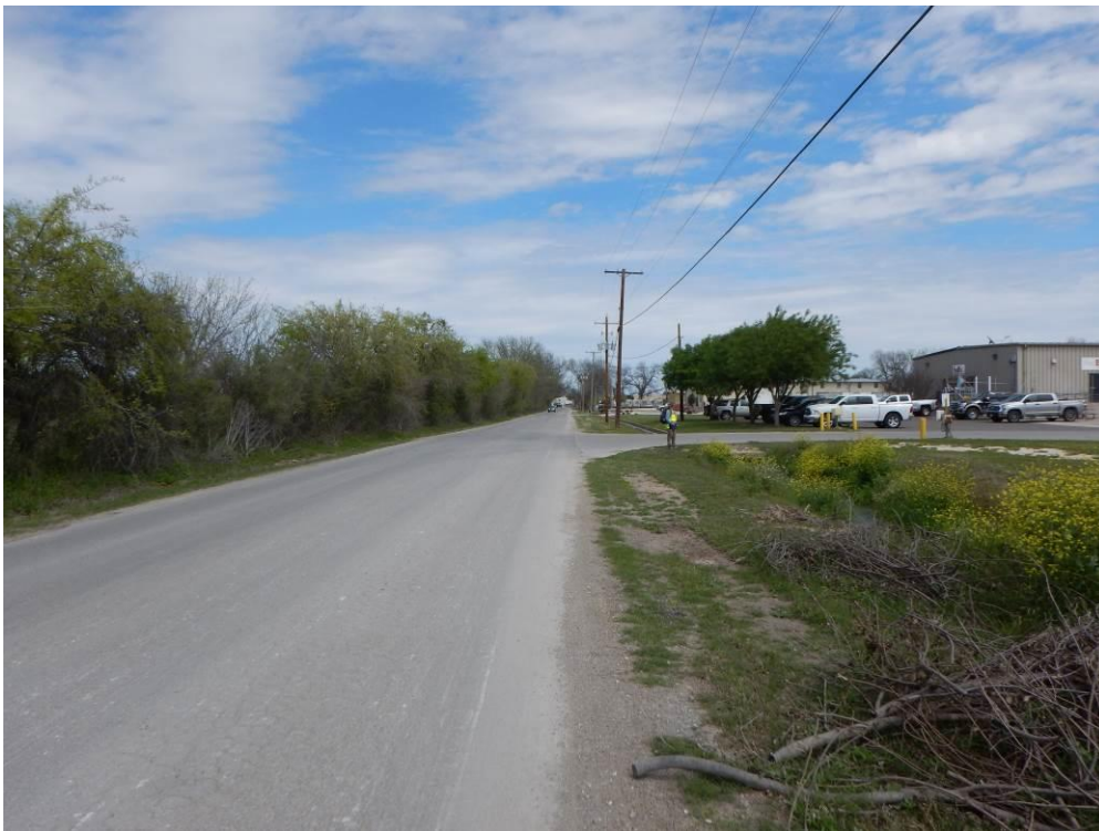
Figure 9. Typical conditions throughout the northern half of the APE: buried utilities within a narrow ROW corridor, paved business entries, and a gravel shoulder, facing north.
