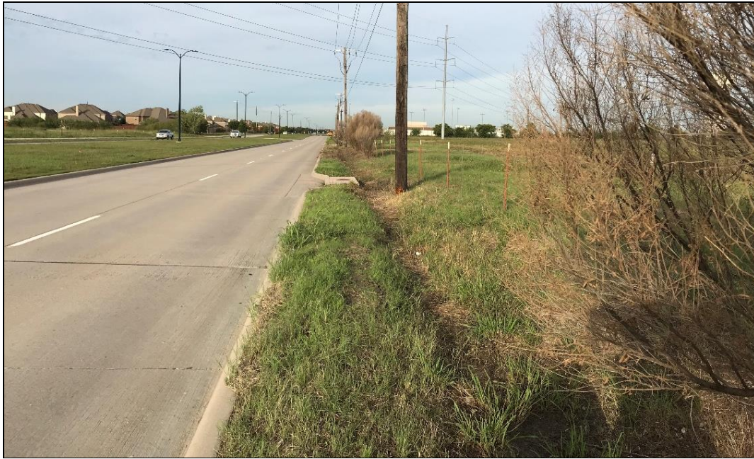
Figure 6. Overview of beginning of APE survey, facing west
