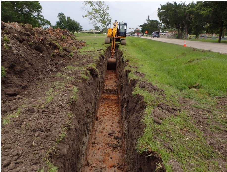
Figure 26. Excavation of Trench 4, facing east. Note distance between roadway and trench.
