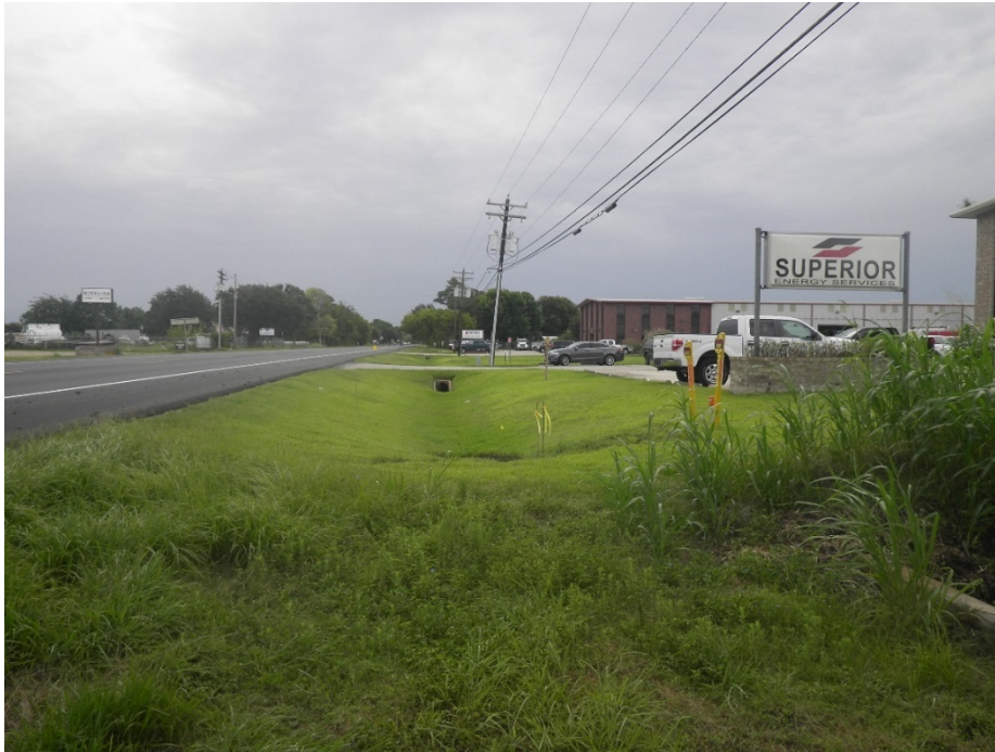
Figure 7. Developed areas south of FM 517, facing east. Note culverts, drainage, and pipelines/utilities.
