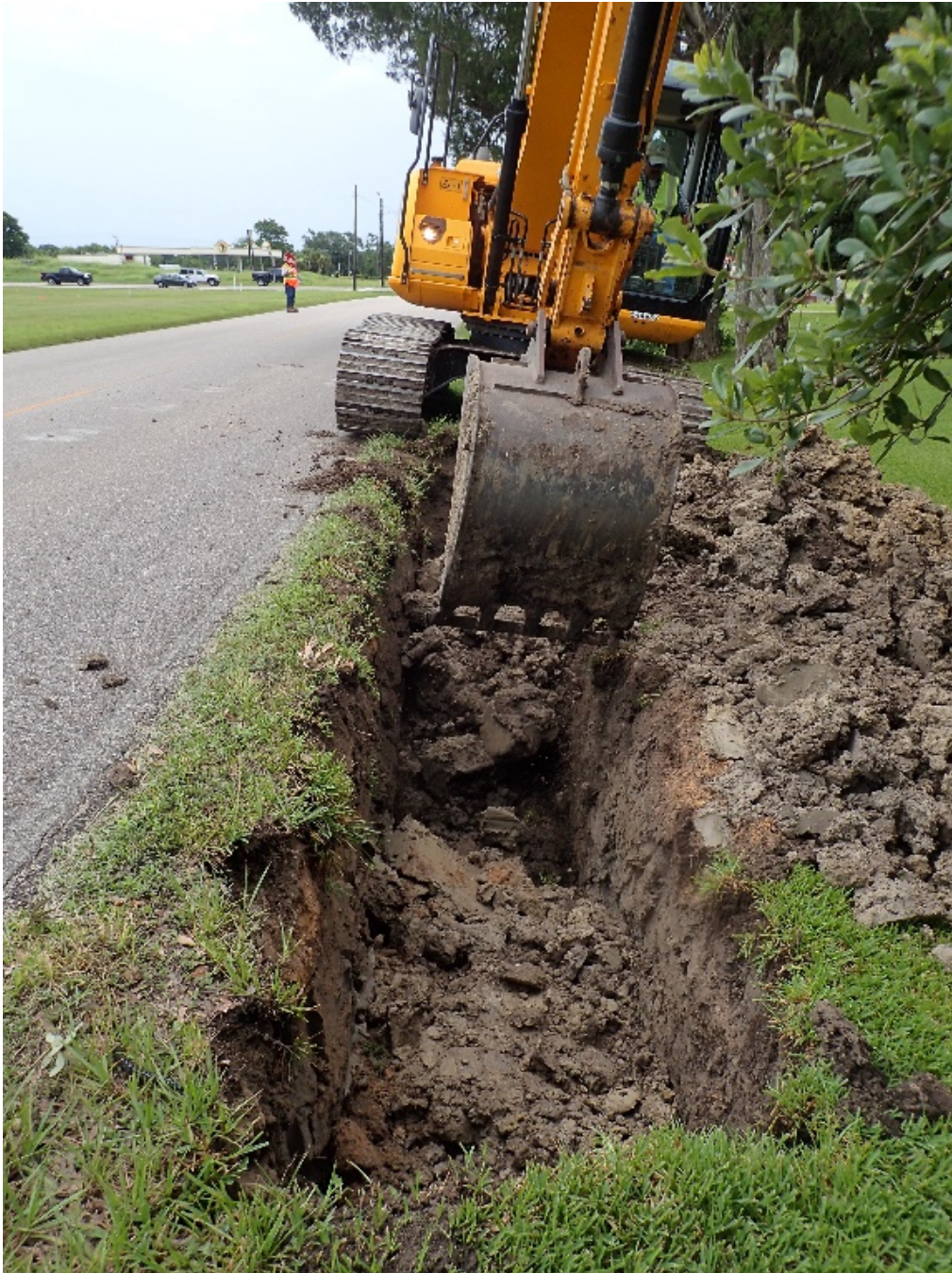
Figure 14. Excavator engaged in trenching, view east. Note proximity to roadway.
