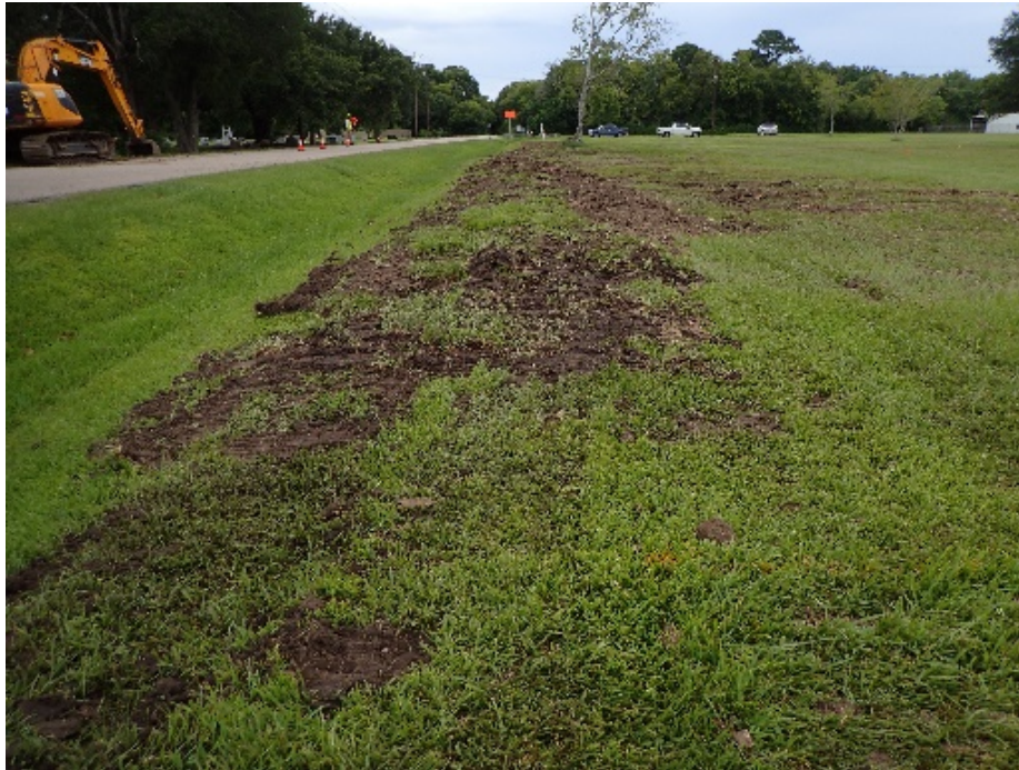
Figure 15. Overview of completed, backfilled trench, facing west.
