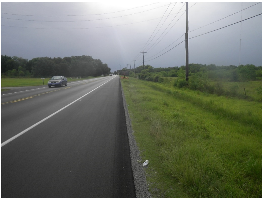
Figure 6. Undeveloped areas south of FM 517, facing east.
