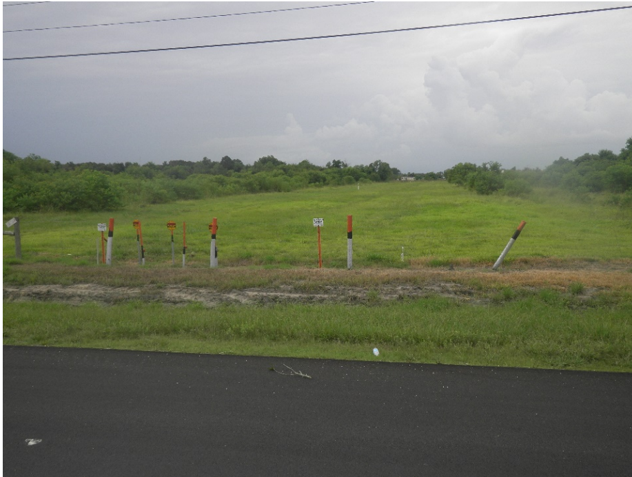
Figure 17. View of oil/gas pipeline development, facing north. Note proximity to roadway and roadway crossing.
