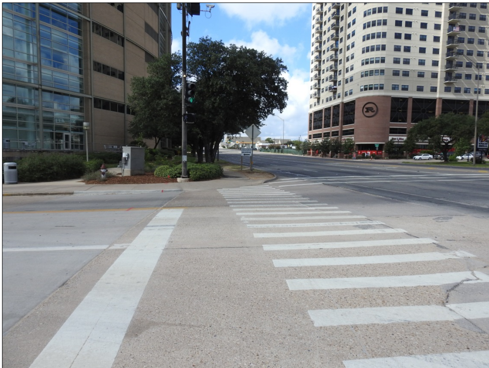
Figure 4-9. Narrow Existing ROW, Paved Surfaces, and Existing Utilities on South Side of University Drive, Facing Southwest.
