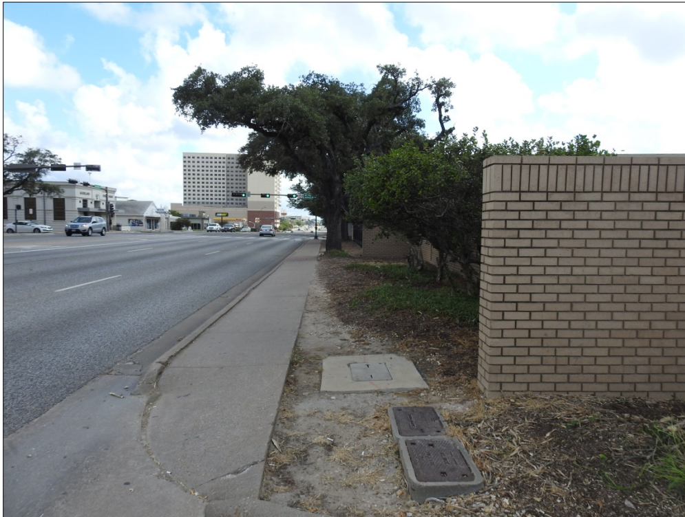
Figure 4-4. Photograph along South Side of University Drive Showing Buried Utilities in a Landscaped Area, Facing Northeast.
