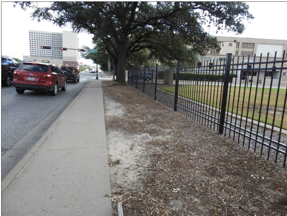
Figure 4-5. Photograph along South Side of University Drive Showing Buried Utilities and Disturbed Soil, Facing Northeast.
