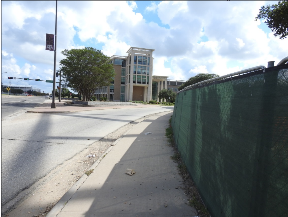
Figure 4-10. Paved Surfaces and Landscaped Median on South Side of University Drive, Facing East.
