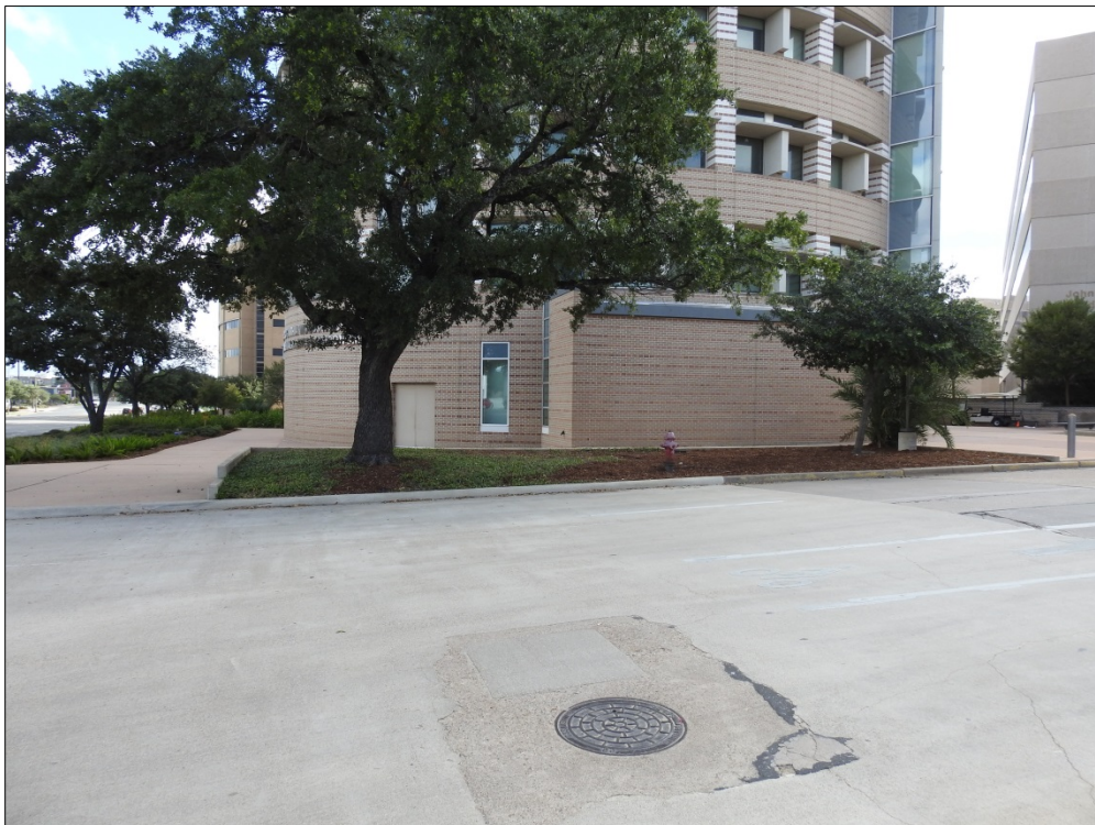
Figure 4-7. Pavement, Sewer Line, and Water Line on South Side of University Drive, Facing Northeast.
