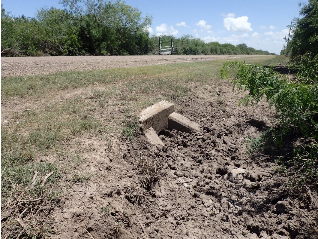
Figure 4-29. HR-05, culvert, west side of culvert, facing southeast
