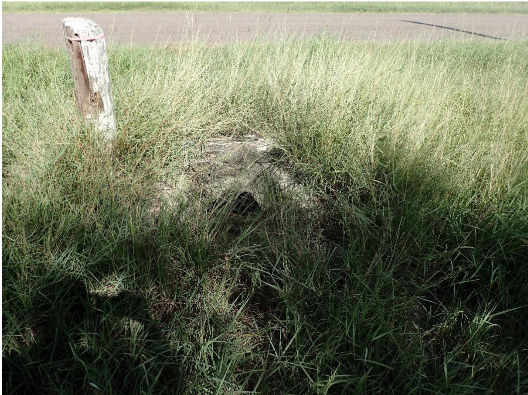
Figure 4-30. HR-06, culvert, east side of culvert, facing west
