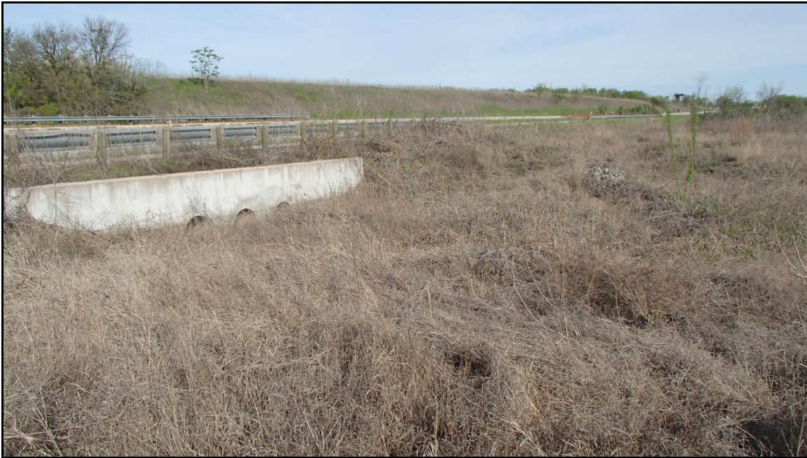
Figure 7: Unnamed tributary of Harris Branch at Howard Lane, facing northwest.
