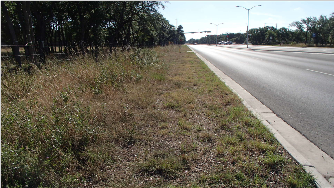
Figure 6. Overview of existing ROW of CR187 near western terminus, facing east
