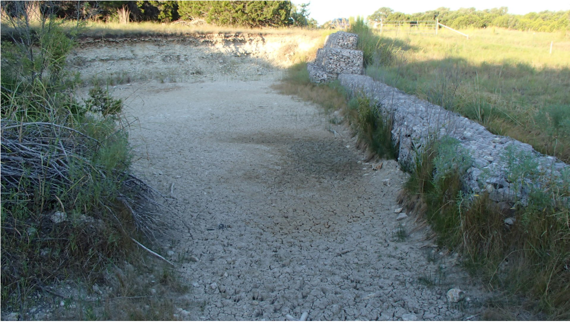
Figure 9. Man-made erosion control feature, facing northeast.
