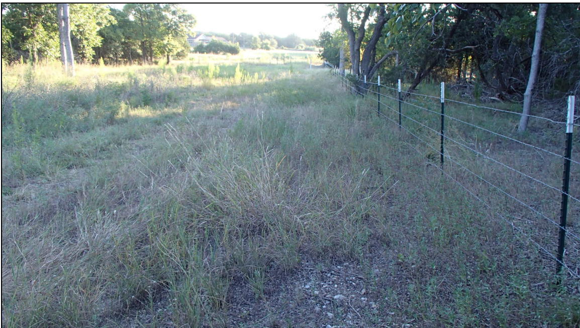
Figure 12: Cleared transmission line corridor, facing east.
