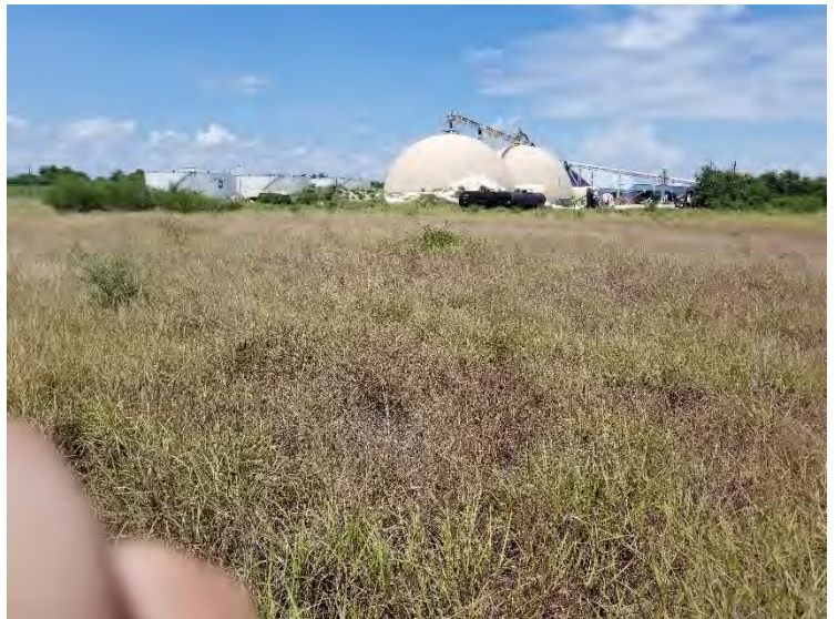
Photograph 12 - Central portion of the APE, view to the north.
