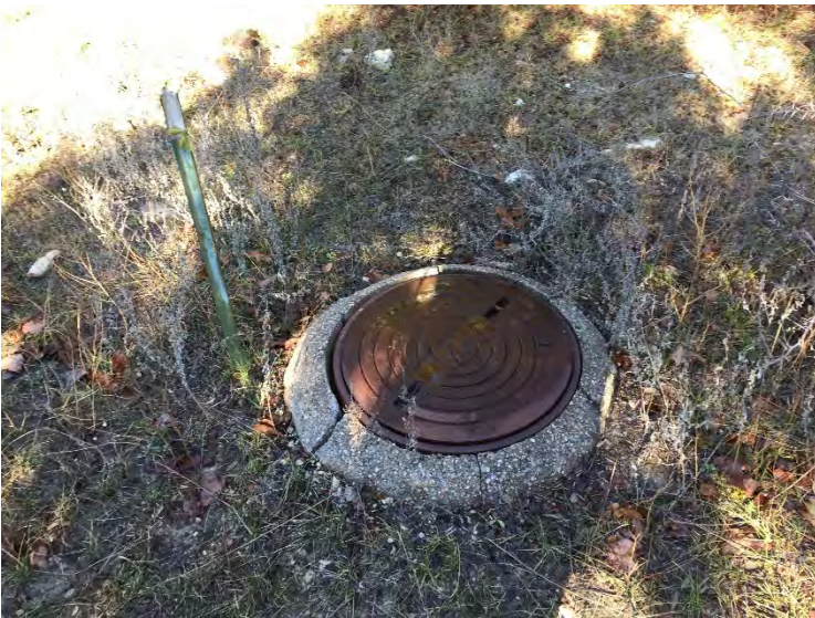
Photograph 15: Modern manhole cover, facing North.
