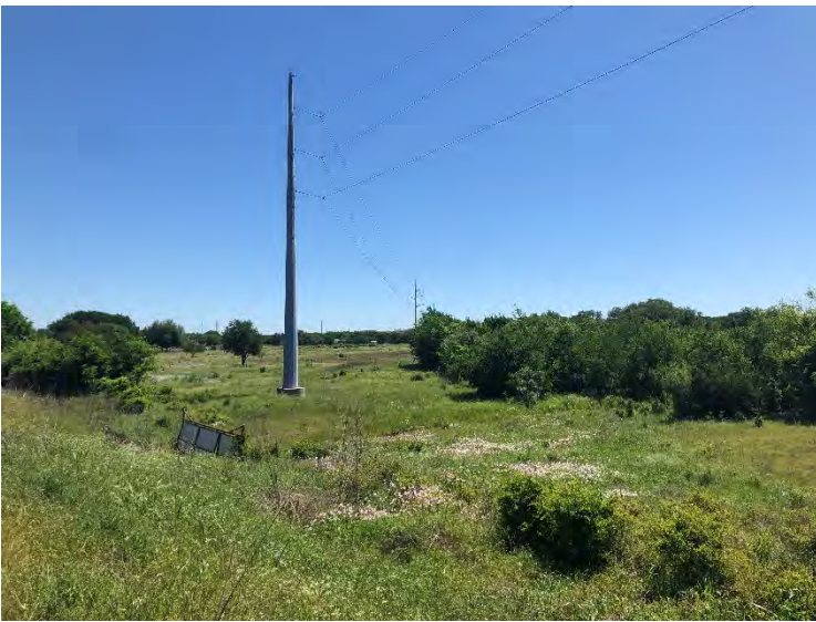
Photograph 1: General APE, utility easement, facing East.
