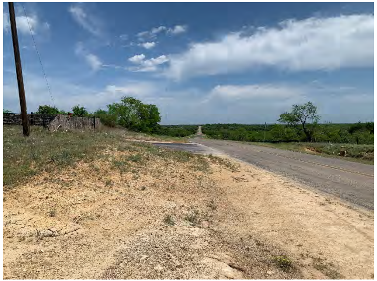
Photograph 32 – FM 3099 ROW, view to the north.
