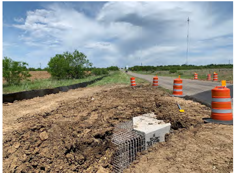
Photograph 30 – Installation of a box culvert under FM 3099, view to the north.
