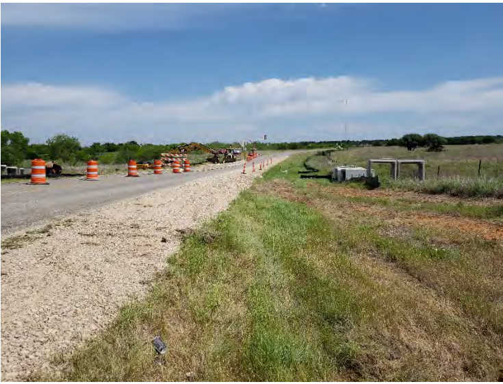
Photograph 25 – Current construction on FM 3099 at Rush Branch, view to the north.
