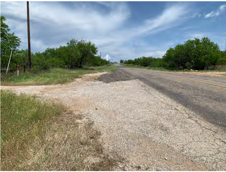
Photograph 31 – Private driveway and FM 3099 shoulder, view to the north.
