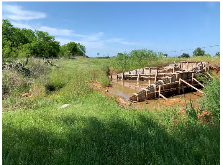
Photograph 8 – Recent drainage construction along FM 2231, view to the east.
