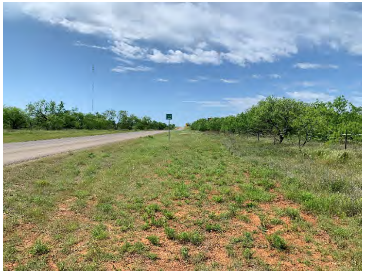
Photograph 34 – FM 3099 ROW, view to the south
