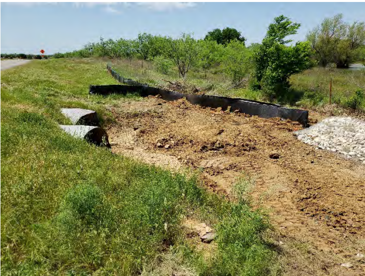
Photograph 29 – Recent rip-rap installation within drainage, view to the south.
