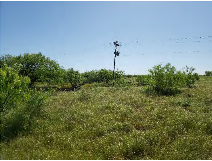
Photograph 43 – Utility line, view to the east.
