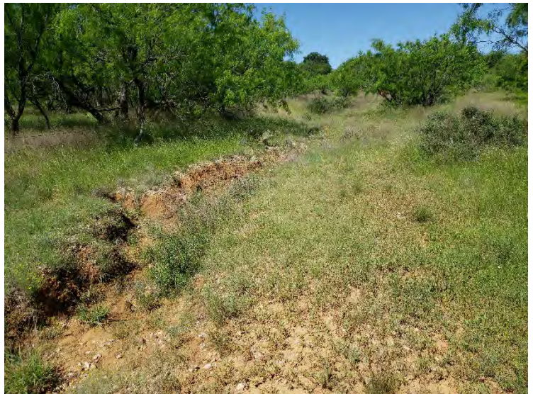
Photograph 48 – Eroded drainage, view to the west.
