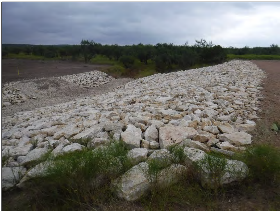
Figure 64. Site 41CX1051 disturbance overview, facing northeast.
