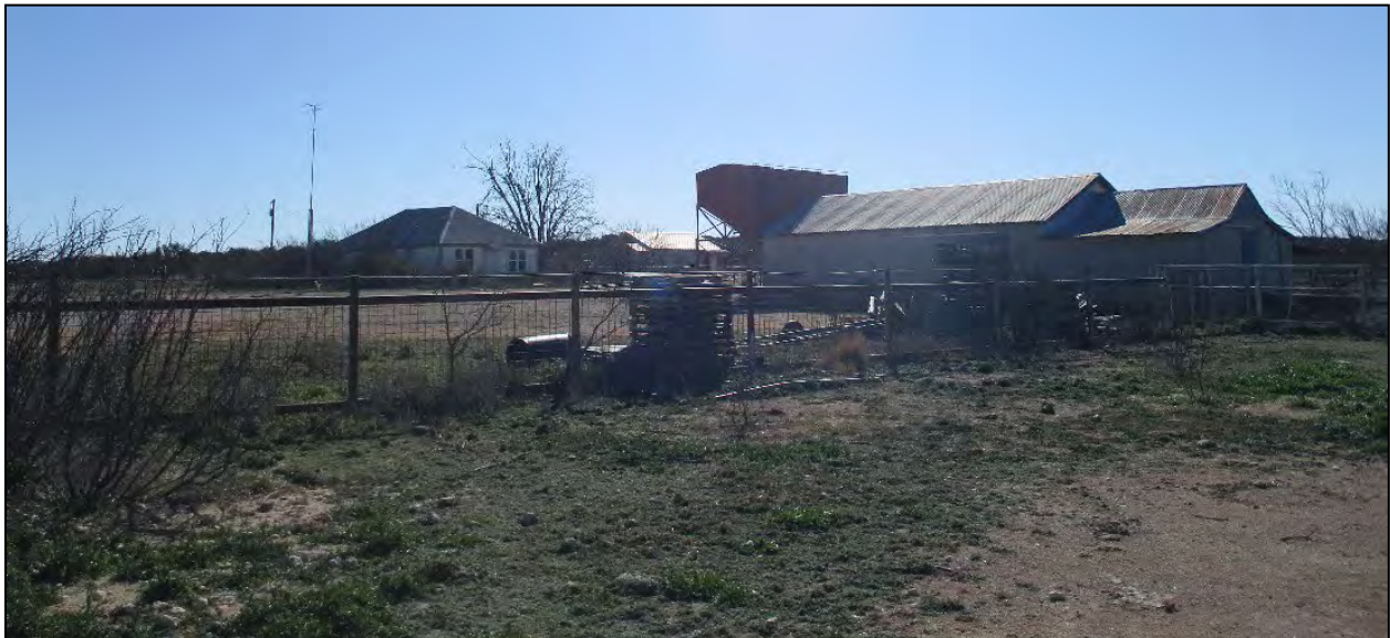
Figure 22. Structures off-site, including house with central passage, facing southeast.
