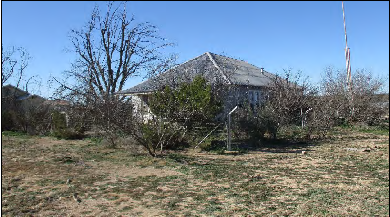
Figure 21. Structure off-site, note ribbon window and hipped roof, facing southwest.
