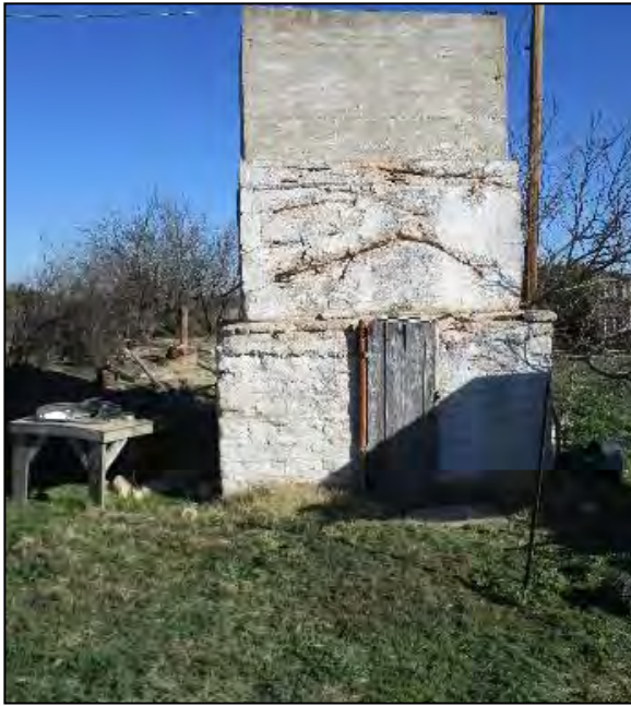
Figure 18. Feature 6 at 41UT147, facing north.
