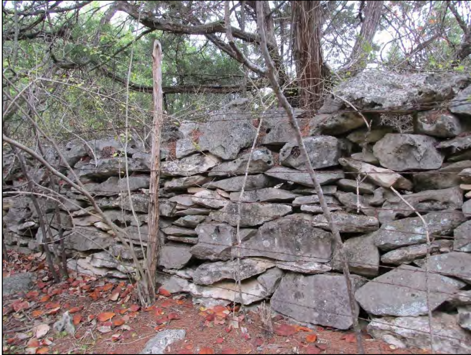
Figure 4. View north-northwest of Site 41WM1416 showing the south façade of the stone wall and the fencing added by the Pooles after 1959 to deter goats from climbing the stone wall and entering the cultivated fields adjacent to Buttercup Creek to the north.
