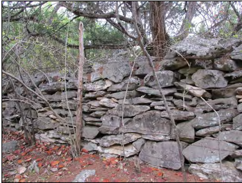
Figure 31. Example of coursing construction, southern façade of rock fence (Freeman 2019)
