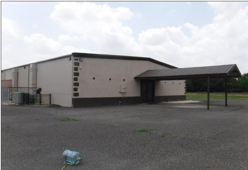
Figure 14. Modern Church in Northern Portion of Project Area (Facing Southwest)
