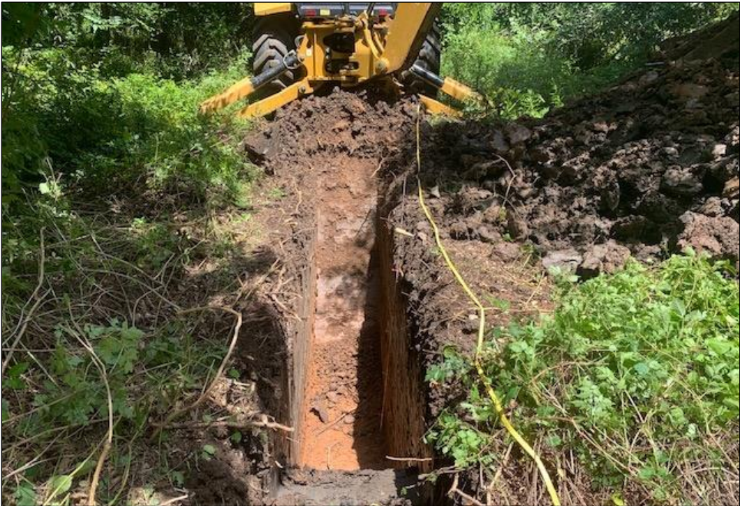
Figure A-9. Overview of BHT-5 (Facing West)
