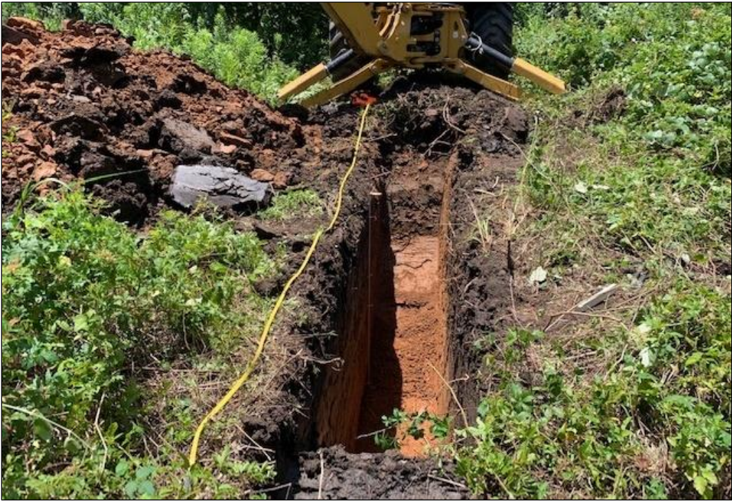
Figure A-7. Overview of BHT-4 (Facing West)
