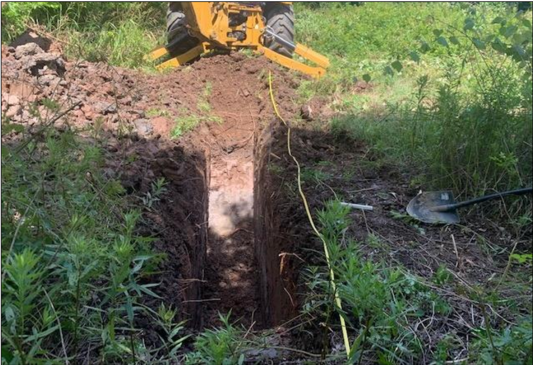
Figure A-11. Overview of BHT-6 (Facing West)
