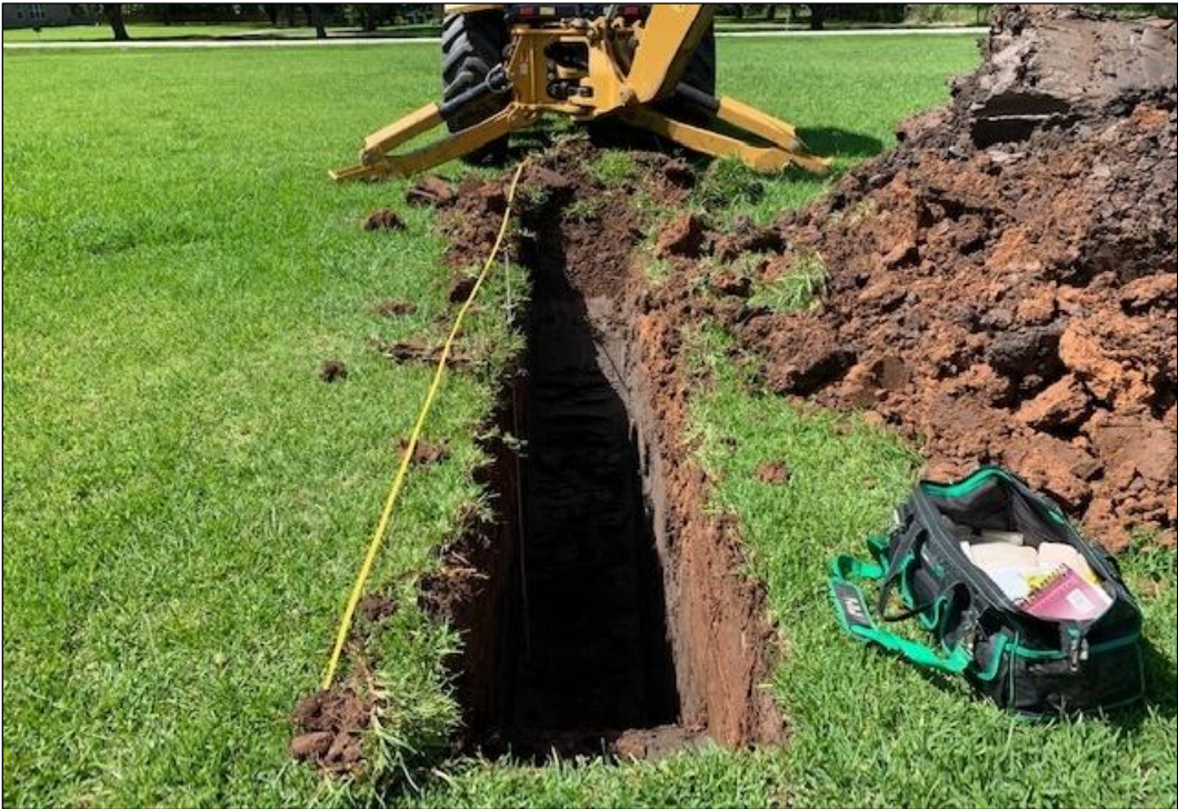
Figure A-13. Overview of BHT-7 (Facing North)
