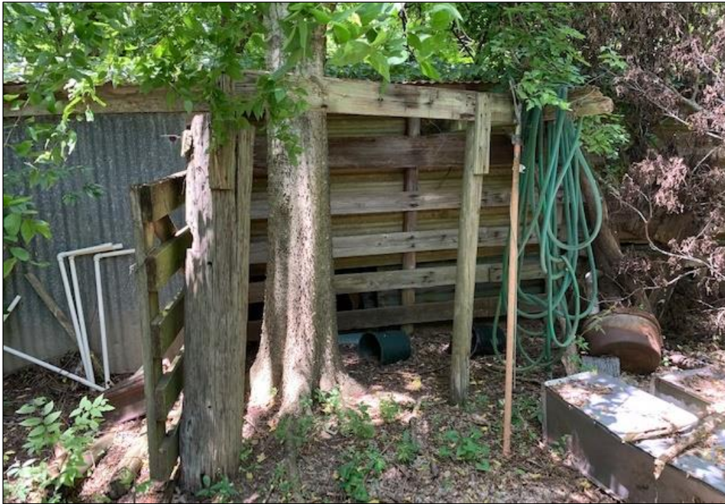
Figure 28. Side of Resource D (Equipment Shed) on Site 41FB365 (Facing North)
