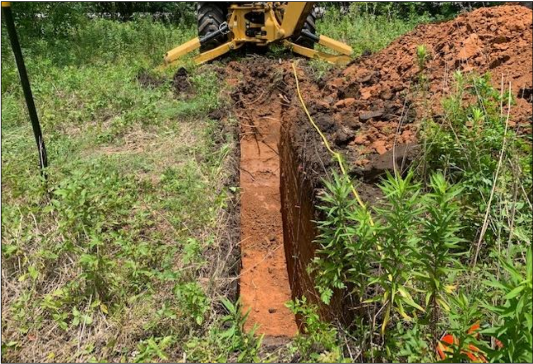
Figure A-5. Overview of BHT-3 (Facing North)
