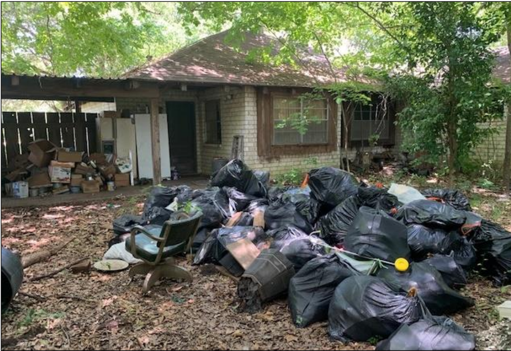
Figure 16. Southern Façade of Resource A (House) on Site 41FB365 (Facing Northeast)
