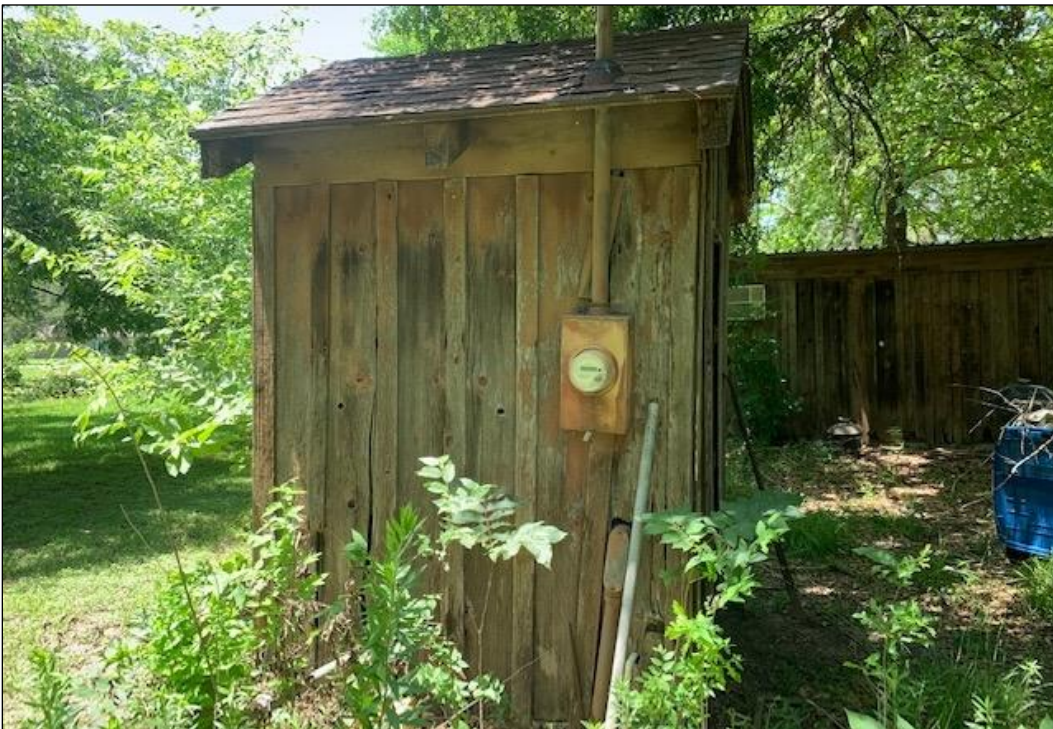
Figure 24. Resource C (Pump House) on Site 41FB365 (Facing North)
