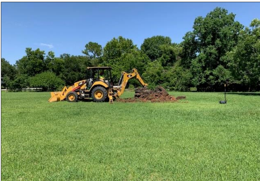
Figure 9. View of BHT07 Excavation Underway within Project Area (East)
