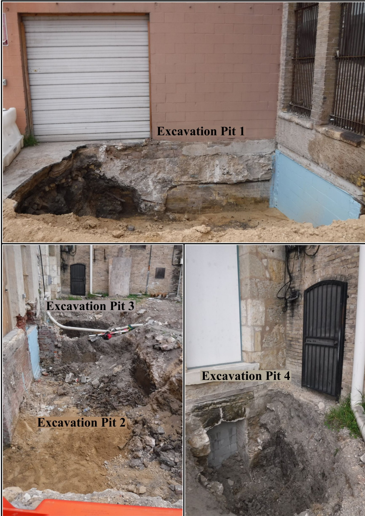
Figure 4-2. Excavation pits at rear of 414 (top), 408 (left), and 406 (right) Dolorosa Street.
