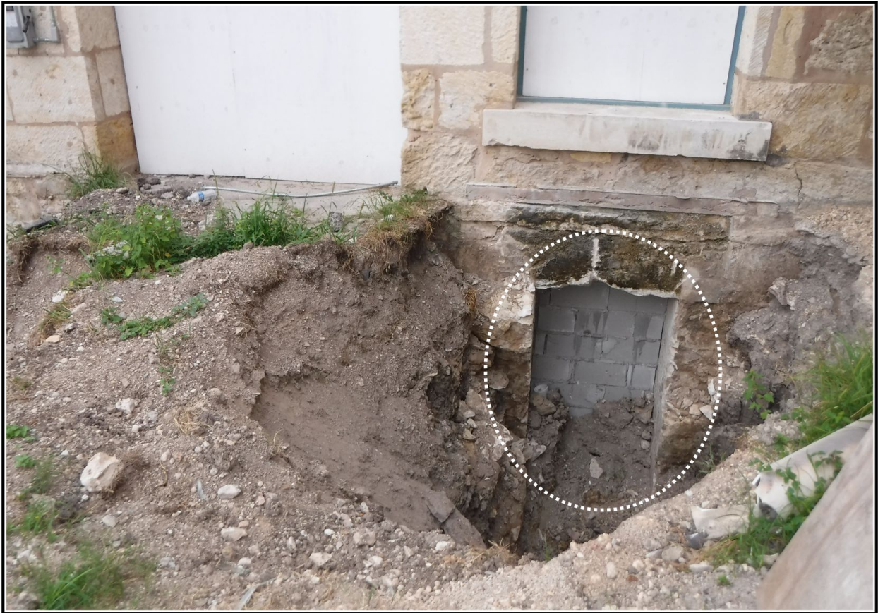
Figure 4-6. Excavation Pit 4 at rear 406 Dolorosa Street; note blocked-off doorway inside pit.
