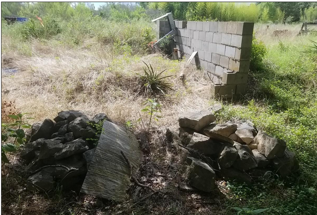
Figure 13. Rock Piles and Cinder Block Wall with Modern Breaker Box and Gas Valve (Facing East-Southeast)
