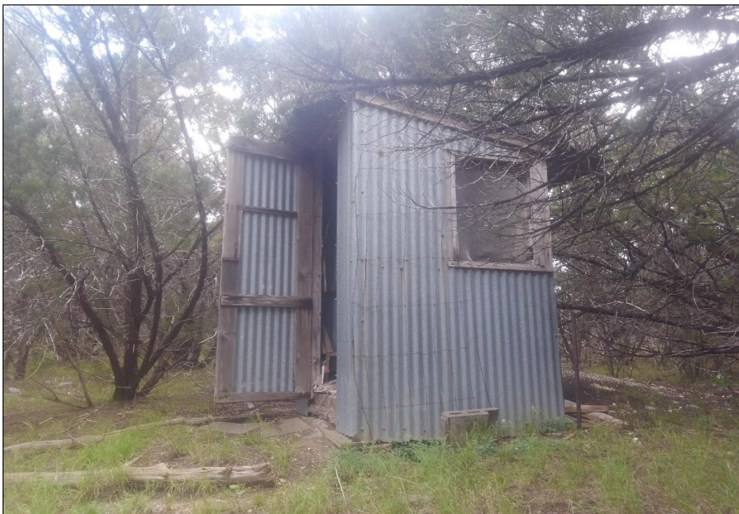
Figure 26. Resource C.1 (Shed) (Facing Southwest)
