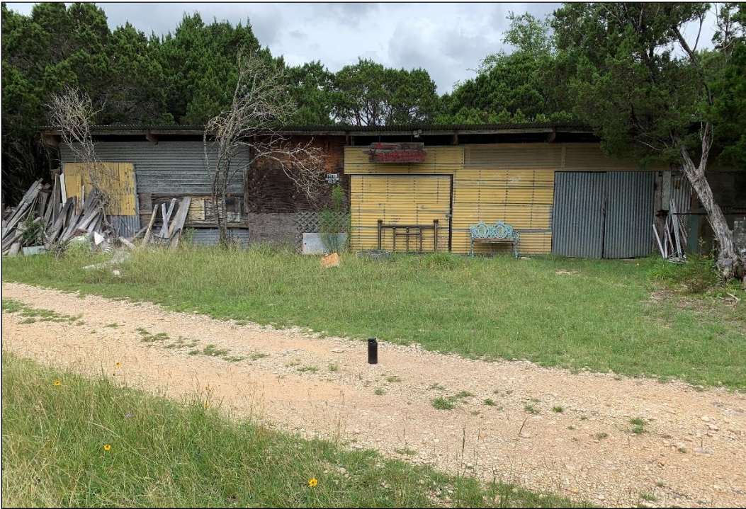
Figure 23. Resource B (Garage/Shed)—Southern Façade (Facing North)
