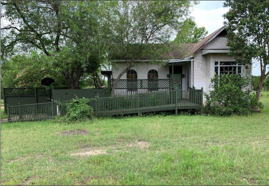
Figure 27. Resource D (House)—Eastern Façade (Facing West)
