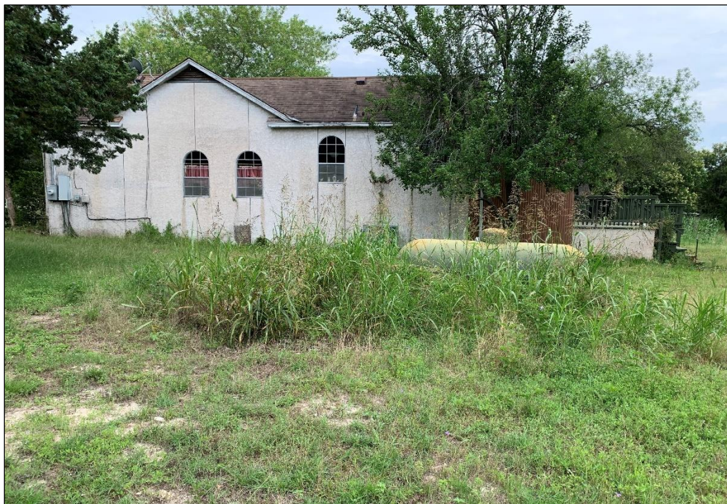
Figure 29. Resource D (House)—Northern Façade (Facing South)
