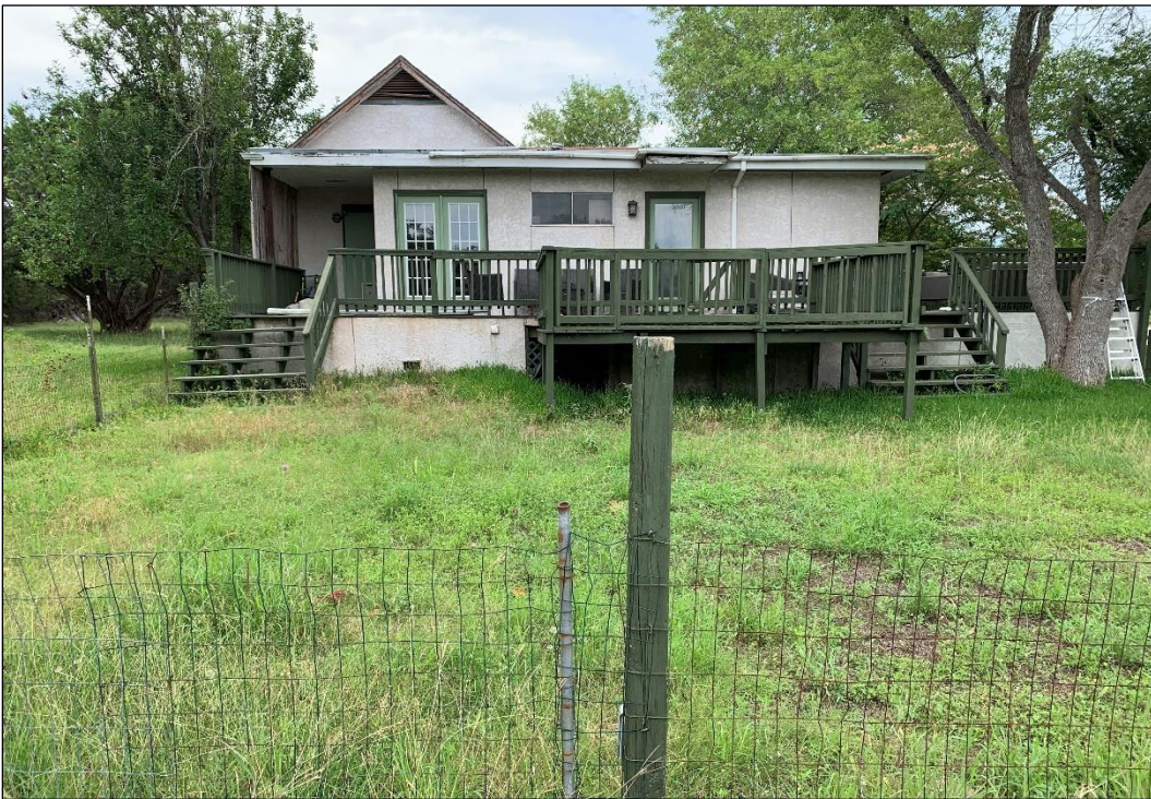
Figure 28. Resource D (House)—Western Façade (Facing East)
