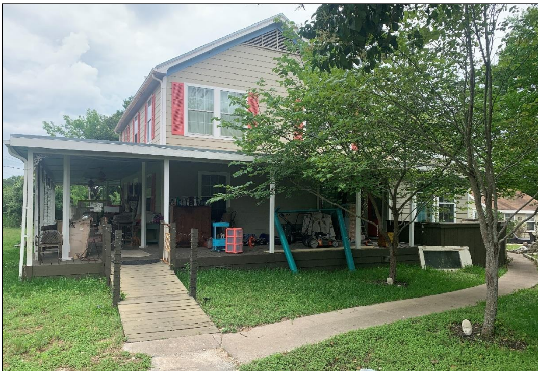
Figure 13. Resource A (House)—Northwestern Façade (Facing Southeast)
