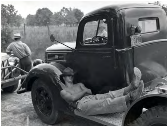
Figure 3-1. 1945 photograph by Esther Bubley of activities in and around 41HR1173.
