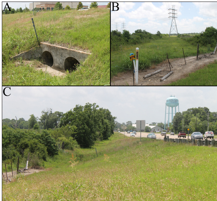
Figure 6.5. Disturbances observed to the north of the HL&P Hot Water Canal and within the APE: A) culvert, photographed facing south; B) pipeline transecting the APE, photographed facing east; and C) artificially raised surface within the APE, photographed facing southeast.
